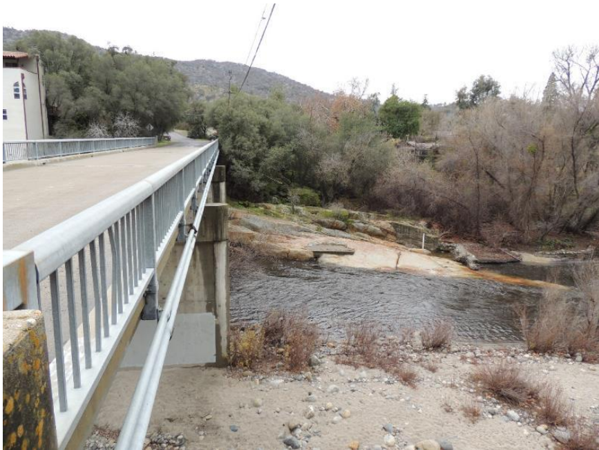
Photo B-20. Dinely Bridge, Downstream Right
