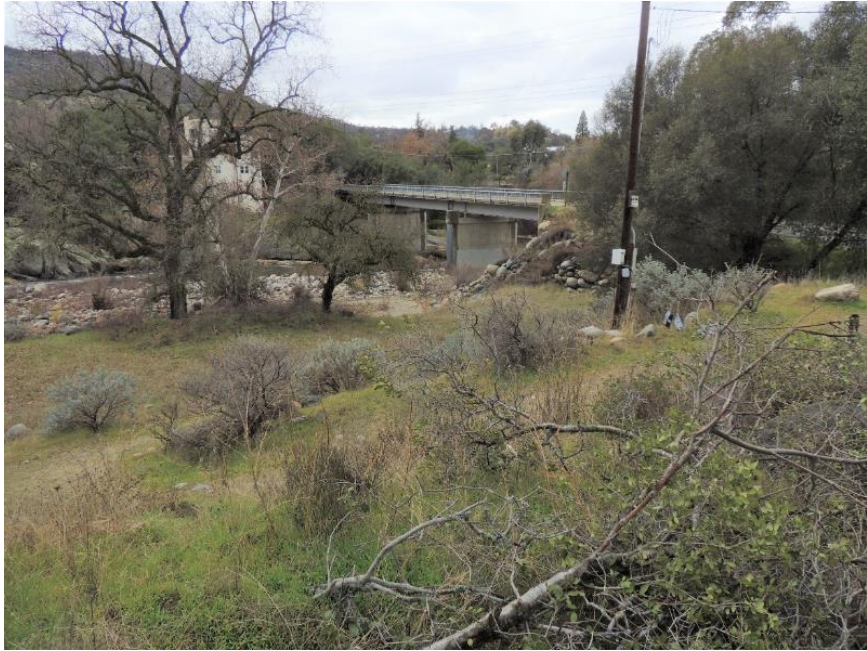
Photo B-21. Dinely Drive, Upstream of Bridge
