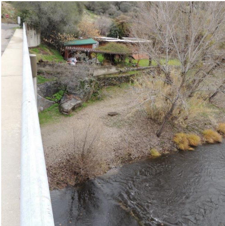
Photo B-33. North Fork Bridge, Downstream Right
