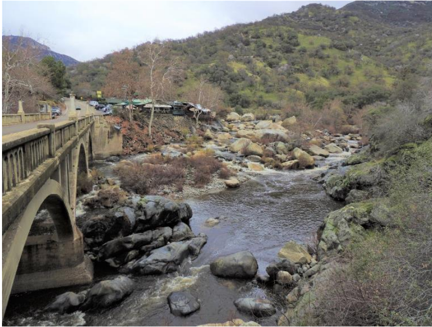
Photo B-7. Gateway Bridge, Upstream Left
