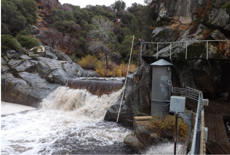
Figure C-5. Image of project barrier at Kaweah No. 1 Diversion Dam. Staff with stadia rod on left bank for scale.
