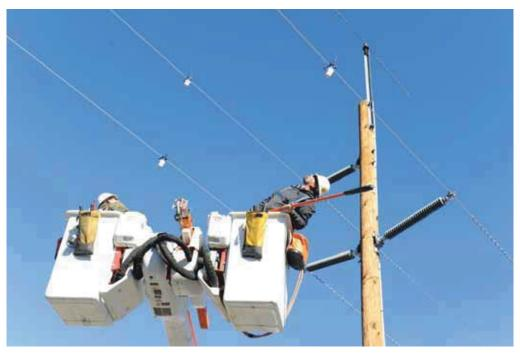
Figure 6. Schweitzer Engineering Laboratories WSO-11 Sensors
