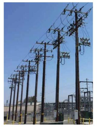
Figure 3. RIS Devices Installed for Site Acceptance Testing
