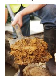
When you call Dig Alert, SCE personnel will come out and mark the pipeline route for you. When excavating near propane gas piping, the excavation must be done with hand tools until the propane gas line is found.
