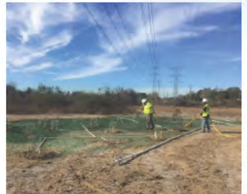
Crews conducting restoration work.
