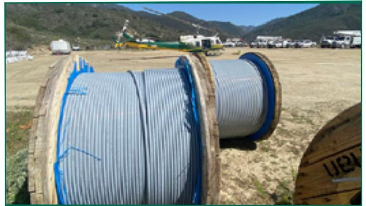
*Covered conductor installation in remote areas can be an intricate process, involving helicopters and dozens of SCE personnel. Photo credit: Casey Wian*
