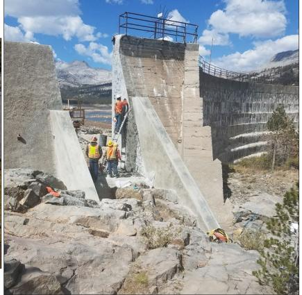
Structural Modifications (2020-2021) – Retrofitted the existing Gem Dam Arch 8 outlet valve to improve hydraulic characteristics of the valve and increase flow releases at the Arch 8 outlet
