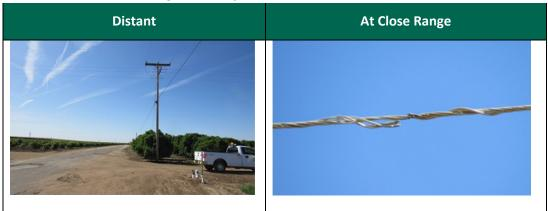
Damaged Primary Conductor on a 12kV Circuit
