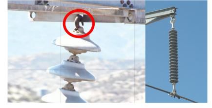
Before-and-After Image of a C-Hook (left) and a New Hardware Replacement (right)
