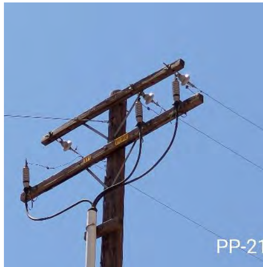
PC-21. Configuration 8: Three-Phase Single-Circuit Undermount
