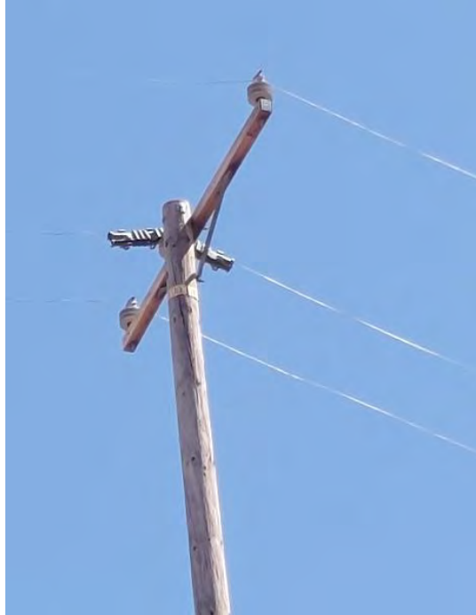
PC-4. Configuration 3: Single-Phase Three-Circuit to Single-Circuit Crossarm
