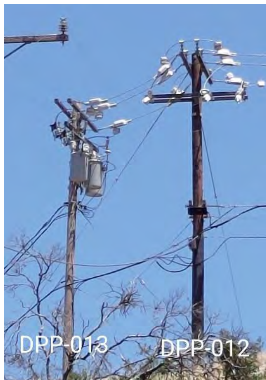
DPP-13. Configuration 11: Three-Phase Transformer Bank
