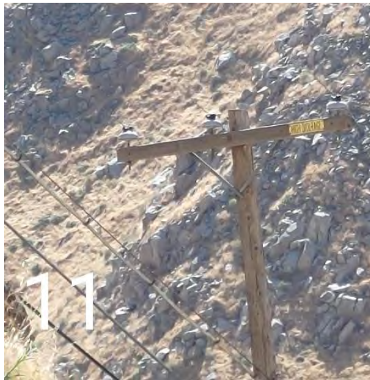
PC-11. Configuration 6: Three-Phase Single-Circuit High Crossarm
