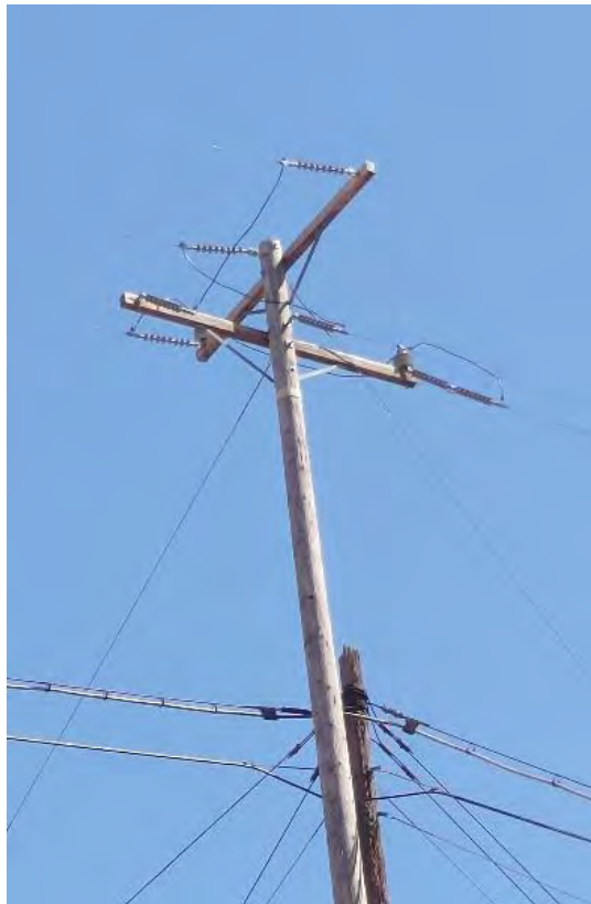
PC-7. Configuration 4: Three-Phase Single-Circuit Dual Crossarm
