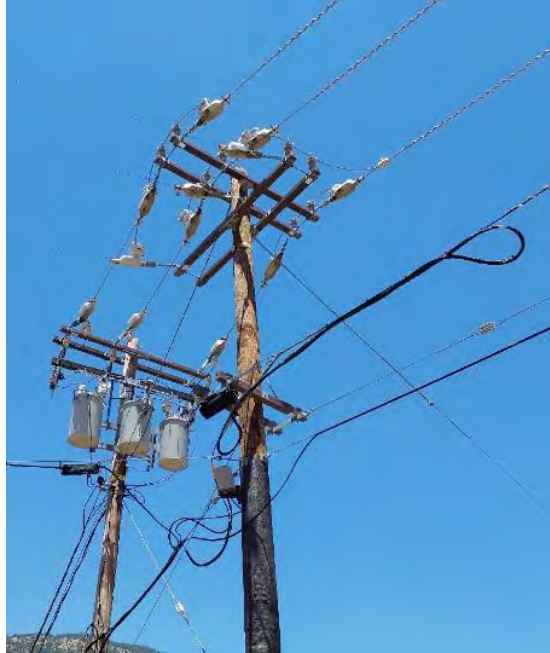
DPP-12. Configuration 10: Three-Phase Distribution Corner
