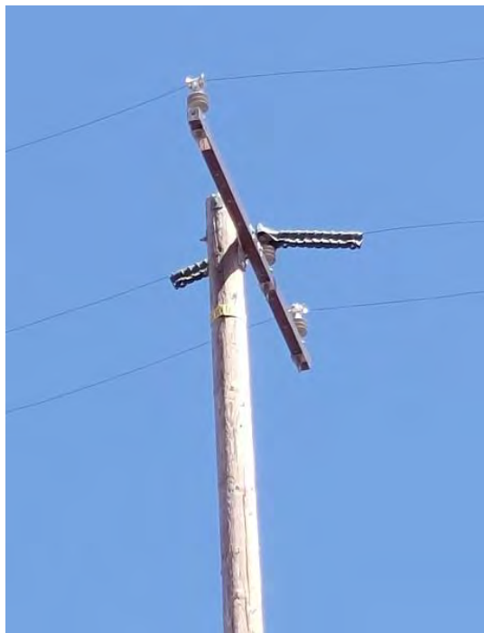
PC-2. Configuration 2: Three-Phase Single-Circuit Crossarm
