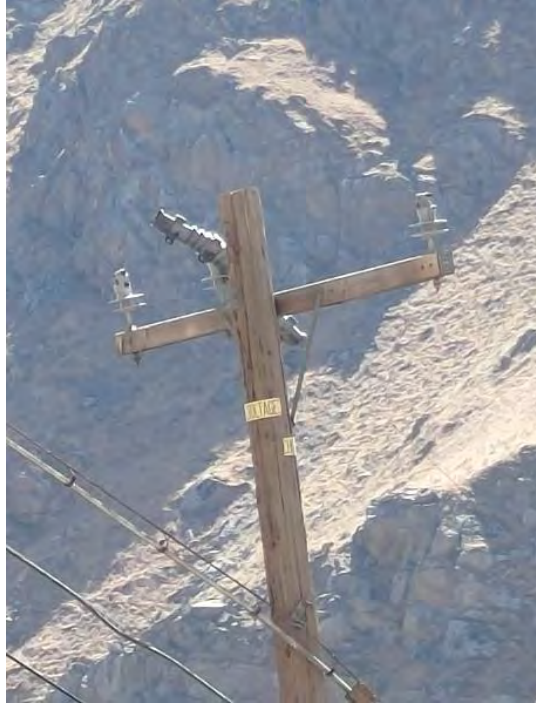
PC-9. Configuration 5: Three-Phase Single-Circuit Low Crossarm
