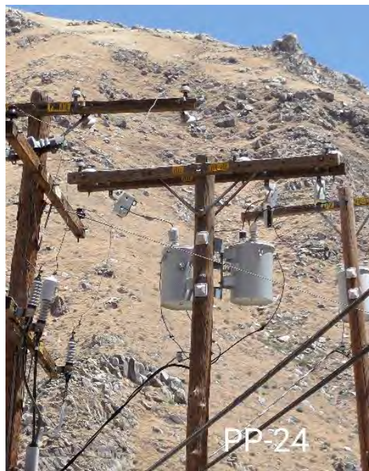
PC-24. Configuration 10: Three-Phase Single-Circuit with Two Transformers
