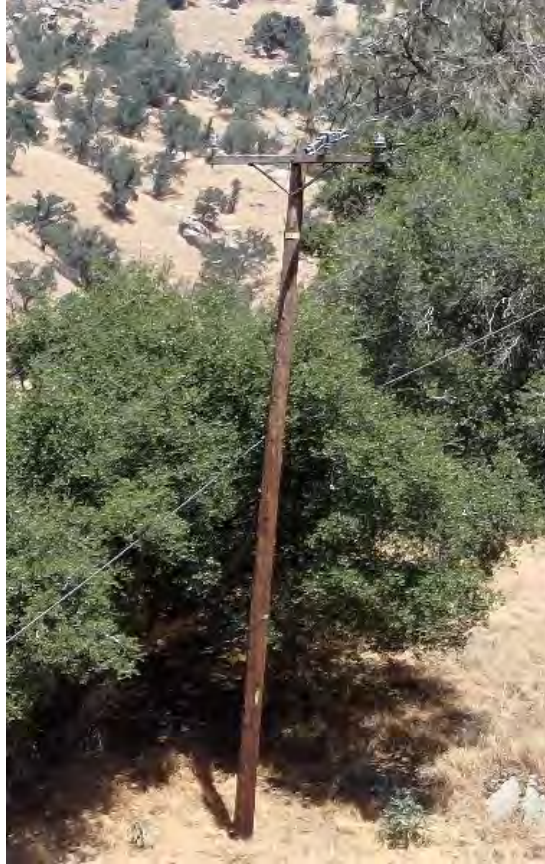
DPP-7. Configuration 7: Three-Phase Single-Circuit Crossarm
