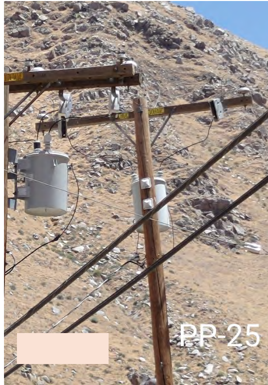
PC-25. Configuration 11: Three-Phase Single-Circuit with Transformer
