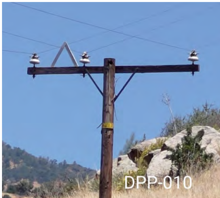
DPP-10. Configuration 9: Three-Phase Single-Circuit Crossarm
