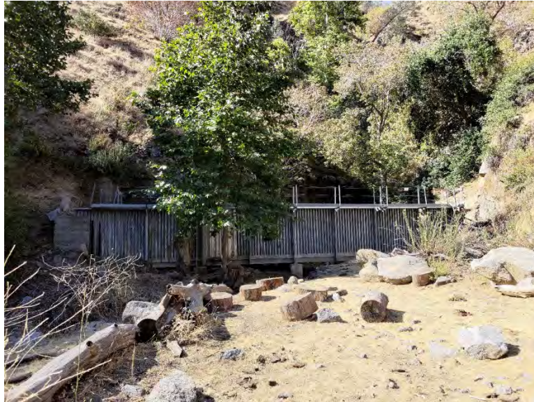
Photo C-10. Stark Creek Area, Flume No. 5 Dougherty Creek: Potentially Accessible to Wildlife. Access to the facility is limited due to the structure's height and metal grate covered walkway. However, open portion of the flume is potentially accessible from the surrounding landscape.
