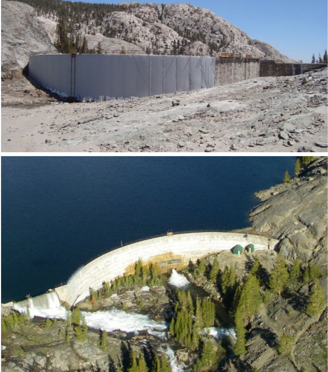
Figure D-11. Rush Meadows Dam photographs showing the bedrock underlying the dam (top = upstream side of the dam, bottom = downstream side of the dam).
