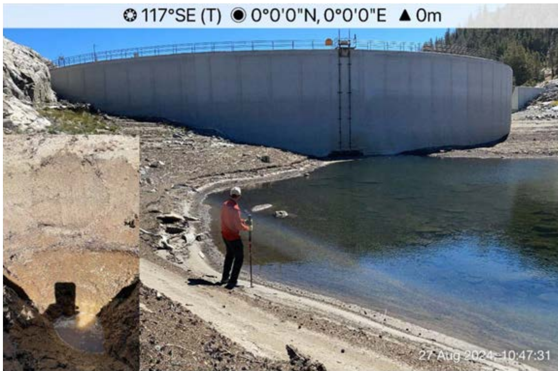
Photo B-11. Waugh 11 contaminant and gradation sample location. Sample pit shows the two visible strata.
