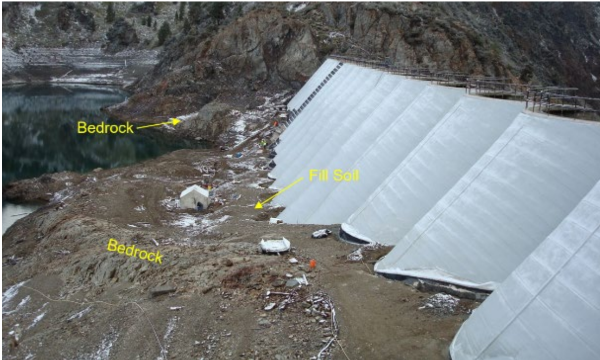
Photo D-1. Photograph taken looking north from the right upstream abutment side of Gem Dam showing what appears to be fill material placed against the dam and within the former outlet channel of the lake.
