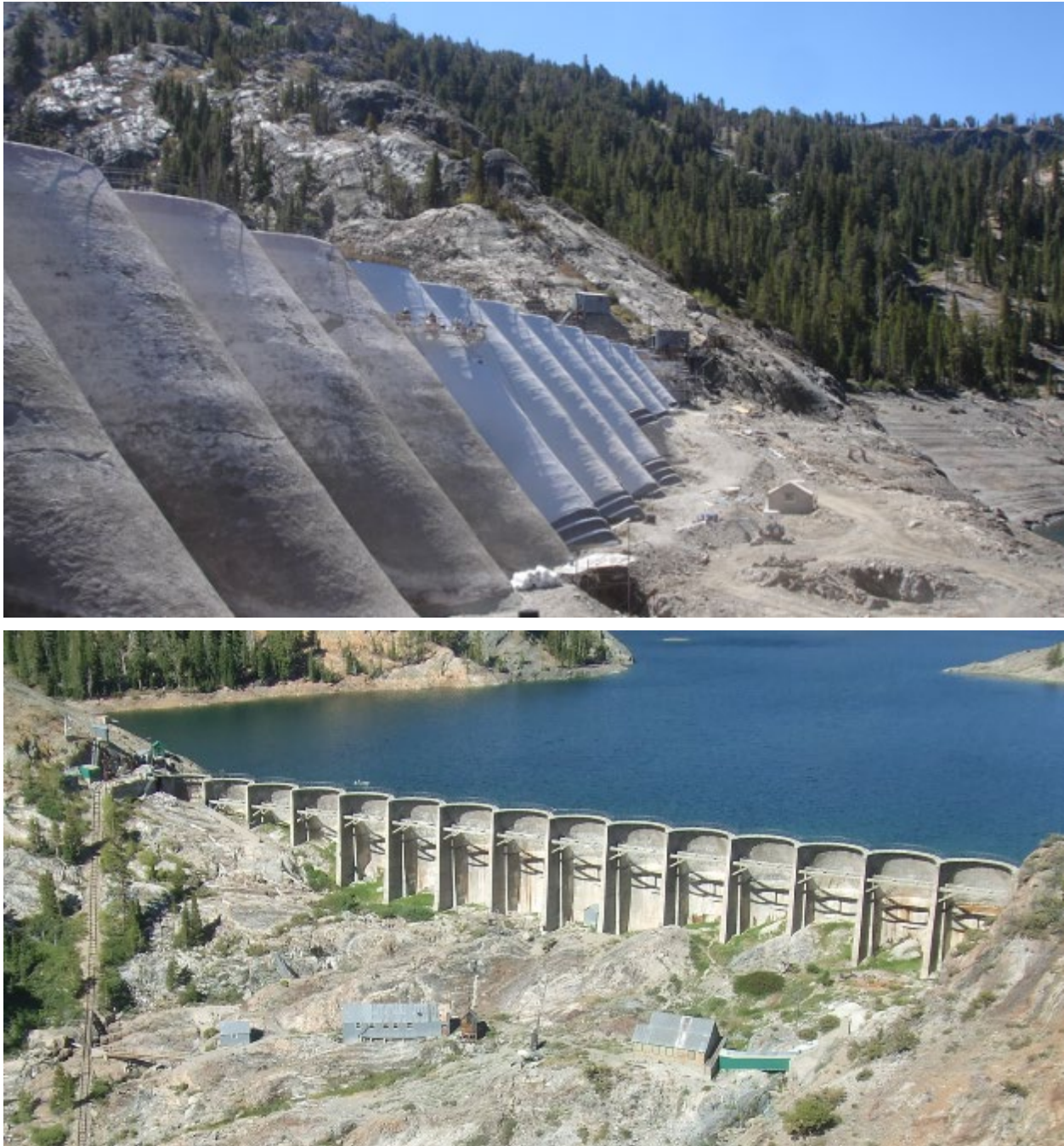
Figure D-14. Gem Dam photographs showing the bedrock ridge underlying the dam (top = upstream side of the dam, bottom = downstream side of the dam).
