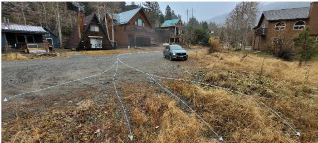
Photo AQ 5-34. Nevada Street surface and inboard ditch runoff diversion with a vegetated buffer between Reversed Creek and the road (location RE-8).
