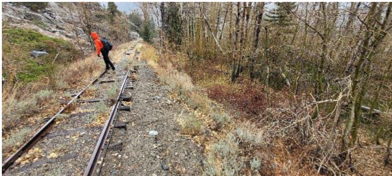
Photo AQ 5-54. Minor surface erosion of the tramway fill slope into a tributary of Rush Creek (location PE-12).
