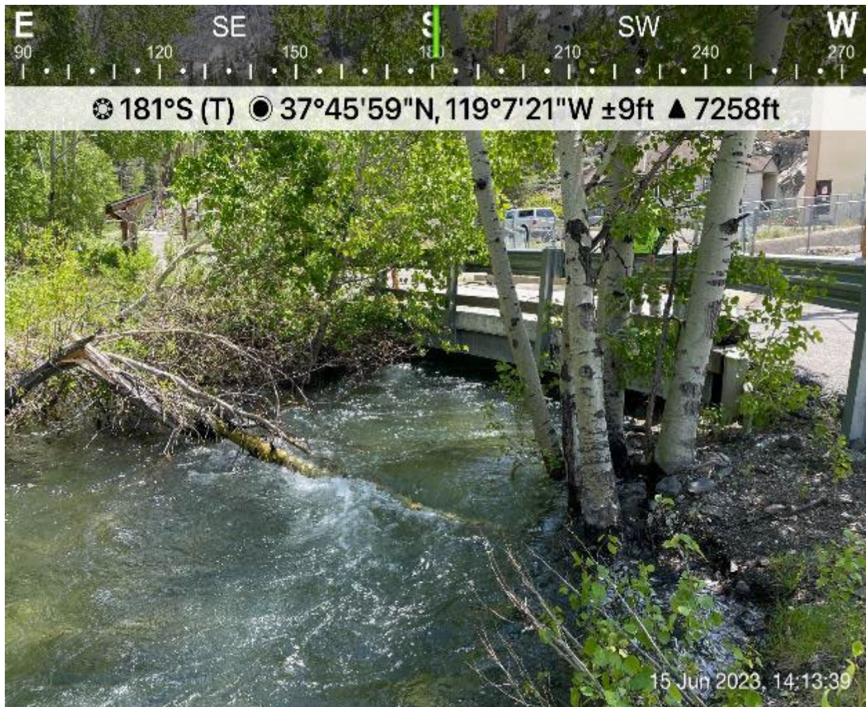
Photo AQ 5-56. Powerhouse tailrace on June 15, 2023. Flow was 106 cfs and sediment concentration was 56.8 mg/L. Channel bottom is visible through clear water.
