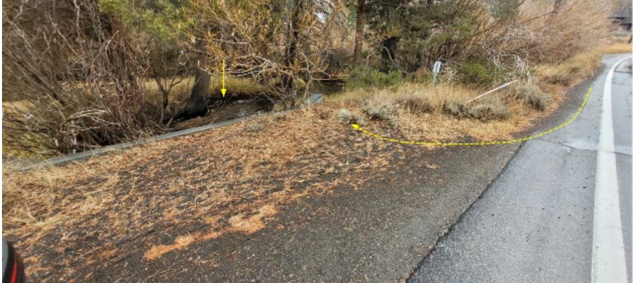
Photo AQ 5-33. Minor sheet and bank erosion associated with the SR-158 Reversed Creek culvert and turnout (location RE-7).
