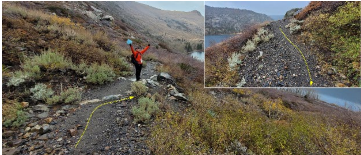
Photo AQ 5-24. Example of a trail runoff diversion structure with minor sediment accumulation due to trail bed surface erosion (location TE-2).
