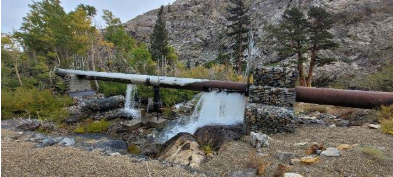
Photo AQ 5-49. Surface erosion and approximately 100 linear feet of gully/channel erosion to Rush Creek from the 2017 emergency cut in the Agnew penstock (location PE-7).
