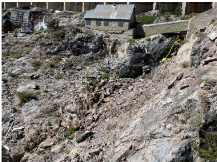
Photo AQ 5-44. Historical erosion of hillslope and drainage below the penstock outlet (location PE-3).
