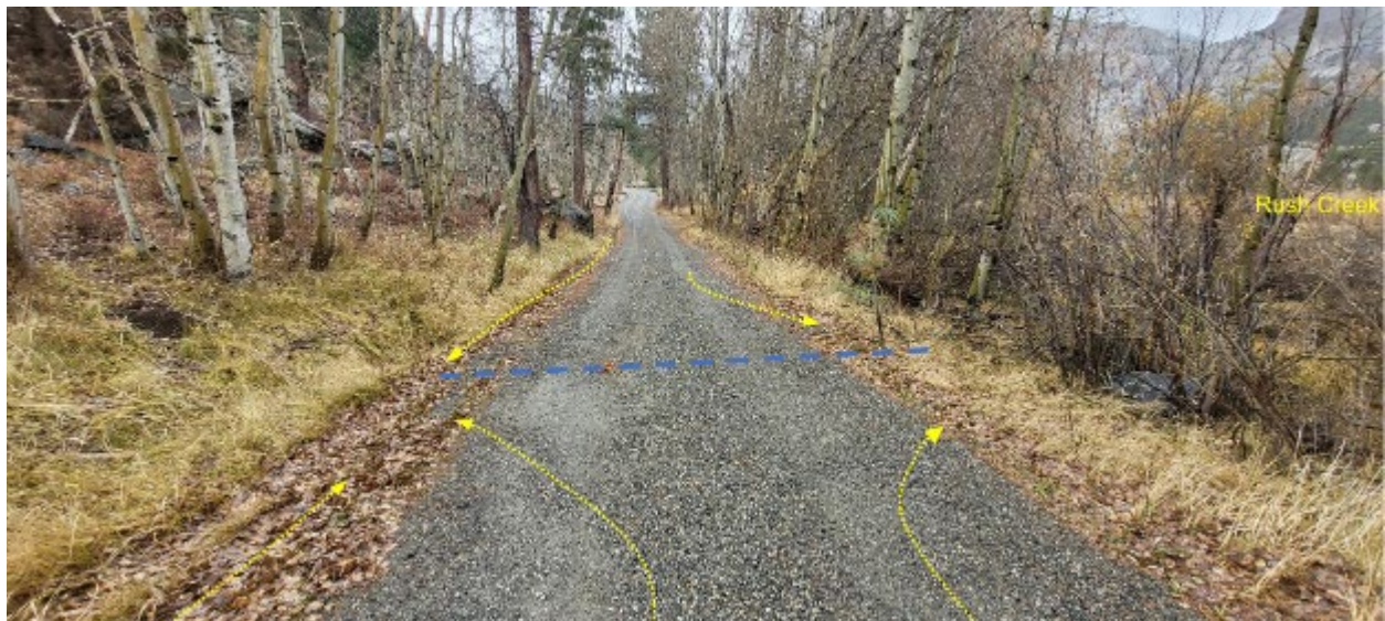
Photo AQ 5-36. Very minor road surface erosion and runoff to a small culvert and large vegetated buffer between Rush Creek (location RE-12).
