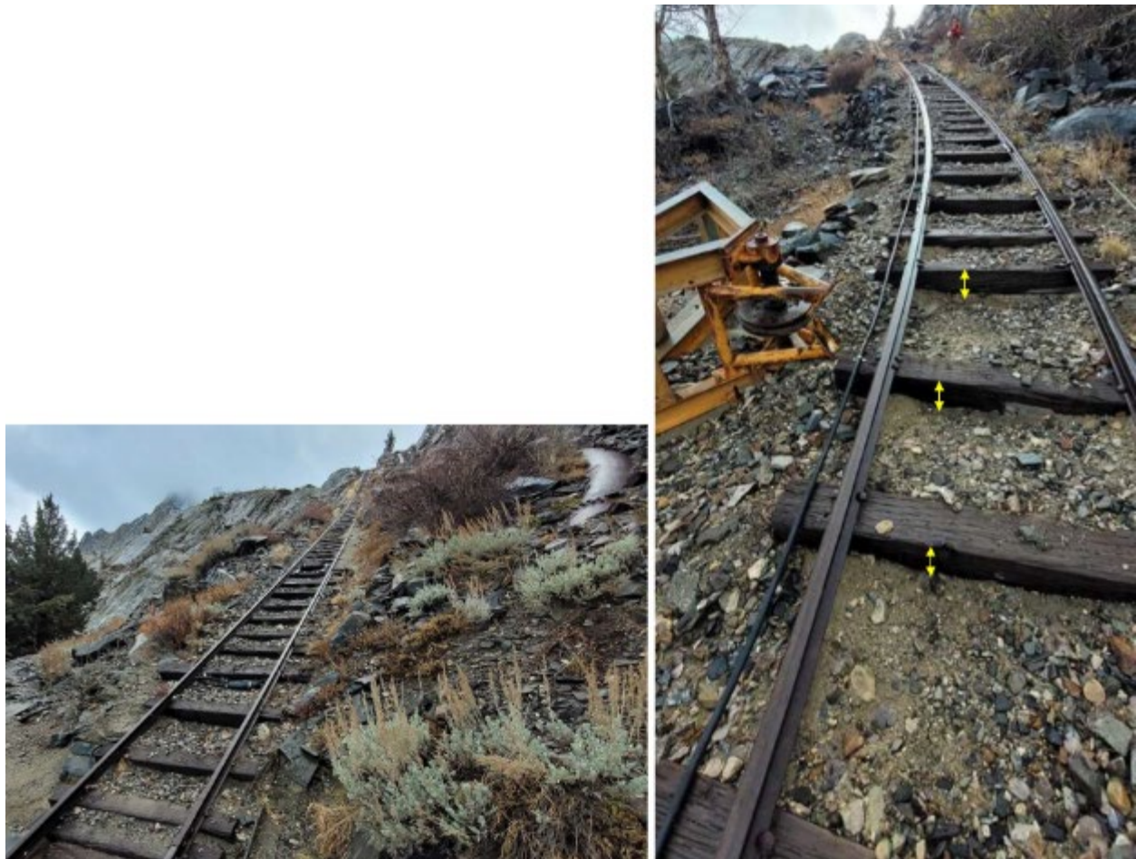
Photo AQ 5-53. Typical surface erosion from around the rail ties in the middle portion of the tramway below Agnew (location PE-11).
