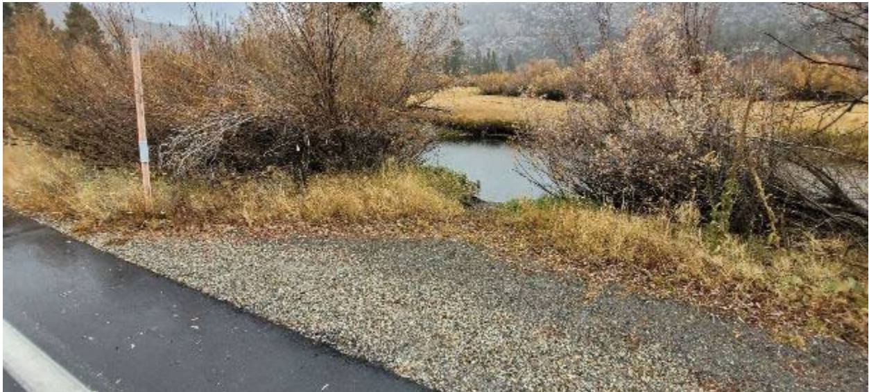
Photo AQ 5-29. Sheet/bank erosion along SR-158 turnout and stream access (location RE-2).
