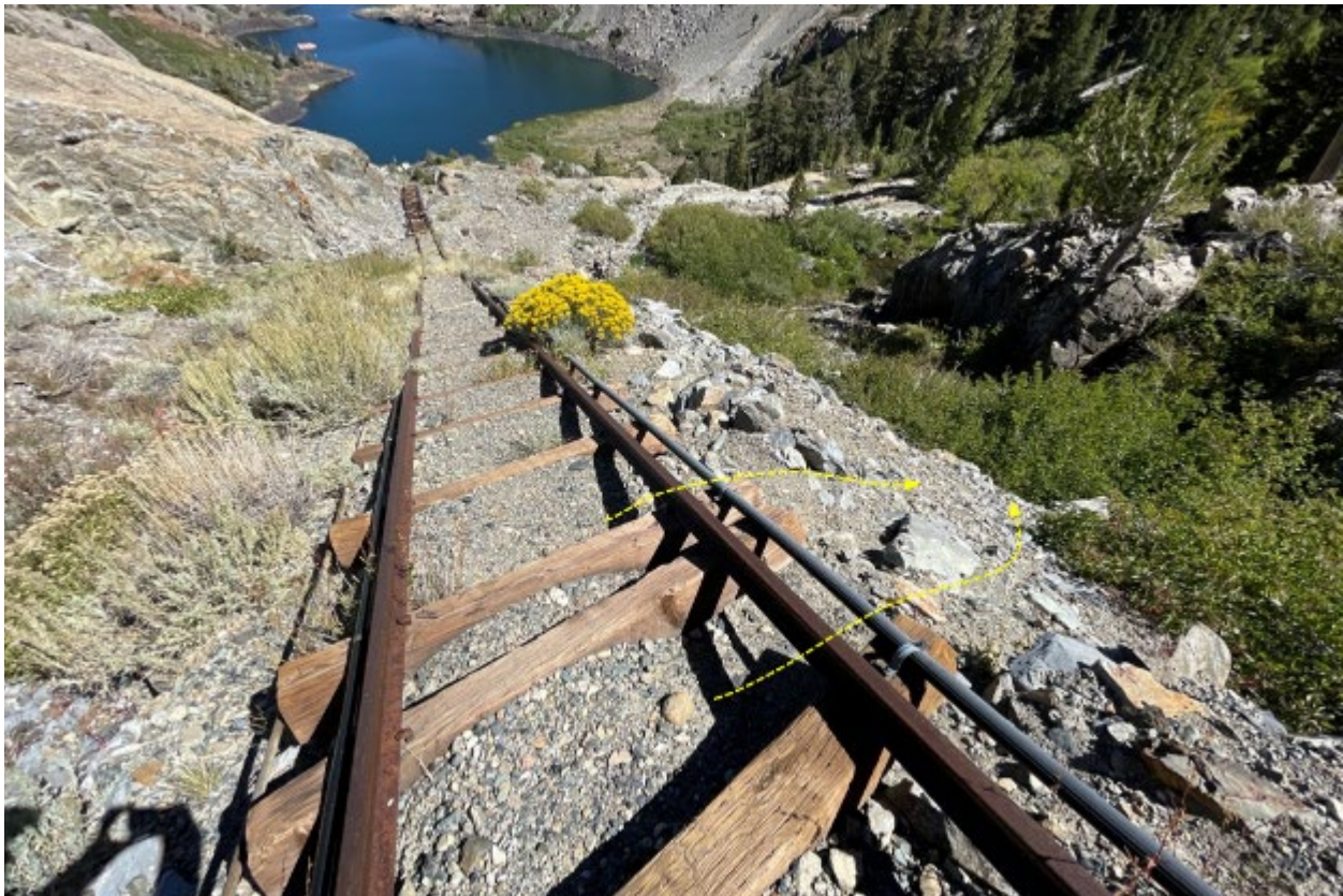
Photo AQ 5-46. Surface erosion from around the tramway rails and fill slope, particularly on steeper pitches (location PE-5).
