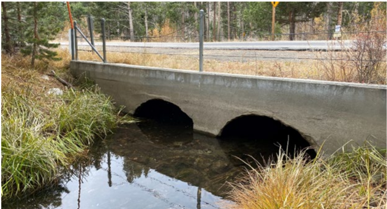
Photo AQ 5-32. Minor surface erosion from the shoulder/turnout at the outlet side of the South Rush Creek SR-158 culverts (location RE-6).
