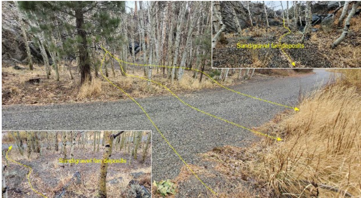
Photo AQ 5-35. Gravel and sand deposition across Nevada Street presumably from a road upslope. Deposition is near a vegetated ditch leading to Reversed Creek, but no indication sediment was transported to the creek (location RE-9).
