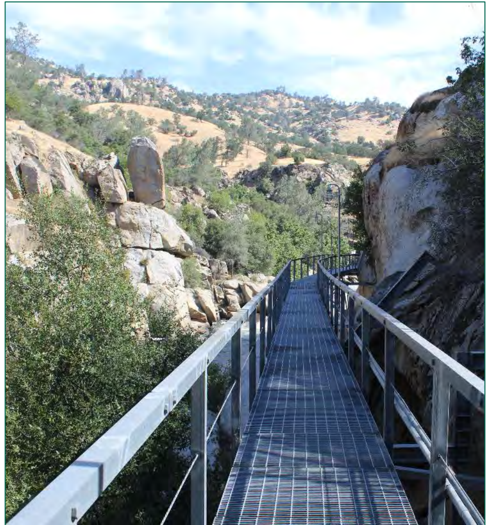
Overview of KR1 Flowline, View North
