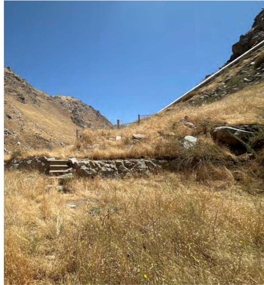
Camp 1, close up of foundation of Building No. 0107 view east.
