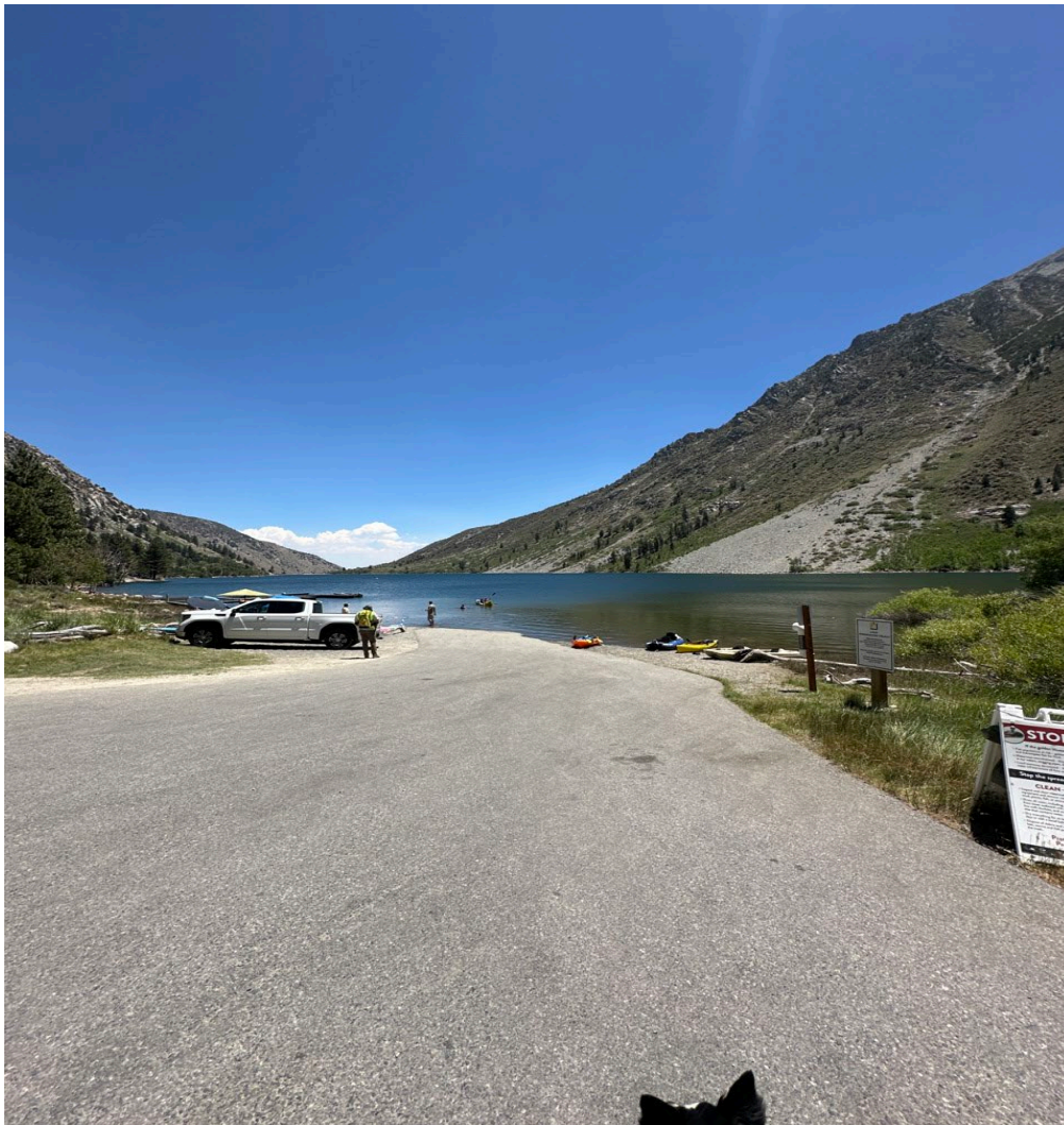
Photo 2-1. Lundy Lake Boat Launch and Parking Area.
