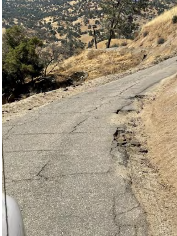
Photo D-3. August 26, 2024. Democrat Dam Road. Example of road surface erosion present throughout this road.
