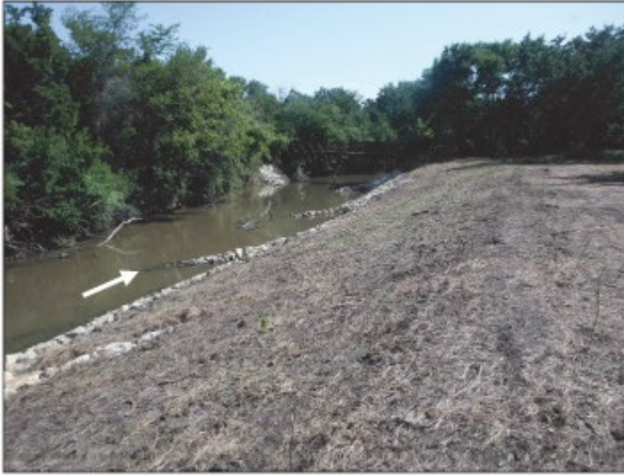
Figure 4-14. Rock Toe Structure
