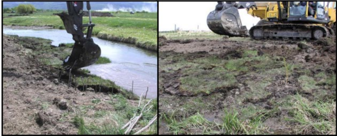
Figure 4-19. Sodmats Placement in a Wetland Restoration Site
