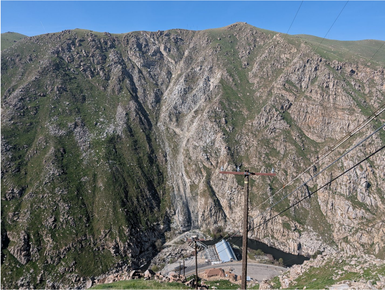
Figure 20. The KR1 powerhouse in the lower Kern Canyon's most scenic and dramatic bend, where large industrial structures and transmission lines are inserted into a High Scenic Integrity Objective landscape. SCE's proposed mitigation for this impact is limited to painting buildings in earth tones. (Photo: Kern Gateway Trail Committee, February 2026)
