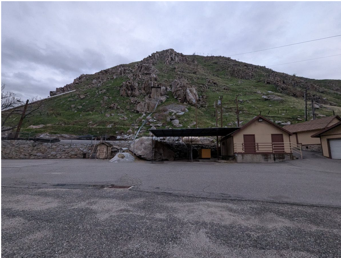
Figure 21. The KR1 Powerhouse parking area — the largest parking lot in the lower Kern Canyon between Bakersfield and Lake Isabella — gated and inaccessible to the public. No trail counter or survey box was installed at this location during the REC-2 study. (Photo: Kern Gateway Trail Committee, February 2025)
