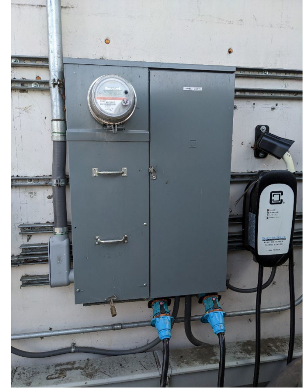
Outdoor Customer Service Electrical Device (CSED) Panel
