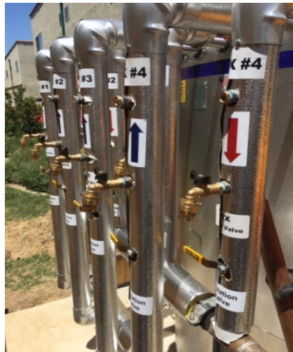
Solar thermal heat exchanger piping
