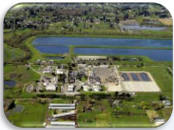
Waste Water Treatment Plant
