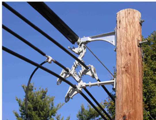
Figure II-6 Spacer Cable Configurations
