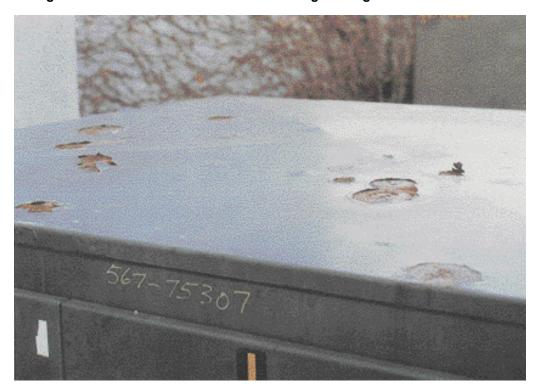
Figure 6–18: Moderate Corrosion with Significant Loss of Paint at Base
