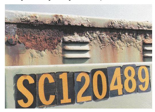
Figure 6–7: Distinct Corrosion of Component Structural Support Members
