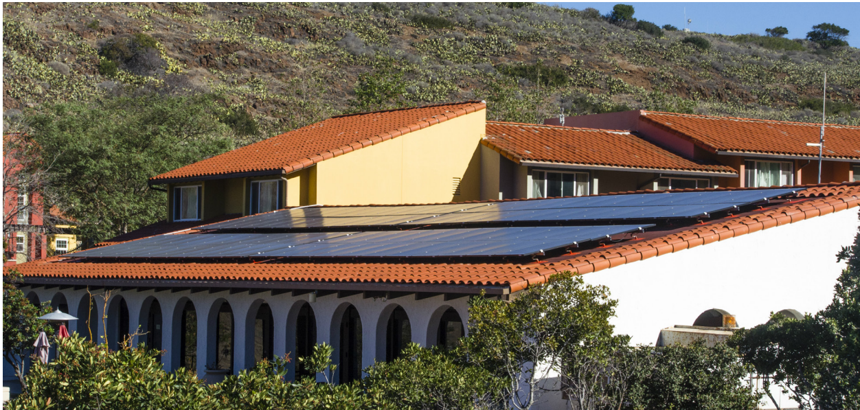
Solar panels at the USC Wrigley Institute for Environmental Studies, near Two Harbors. Credit: Karl Huggins/USC Dornsife
