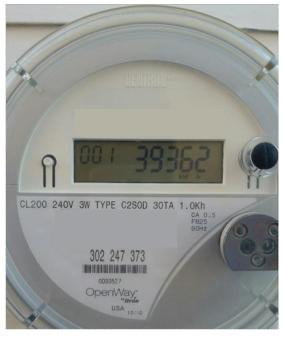
Channel 001: Displays total kwhs usage since meter was set. Similar to car's odometer, the counter increases by 1 every time 1 kWh (1000 watts) is used. It does not reset but dials over after 999,999 kWh have been captured.
