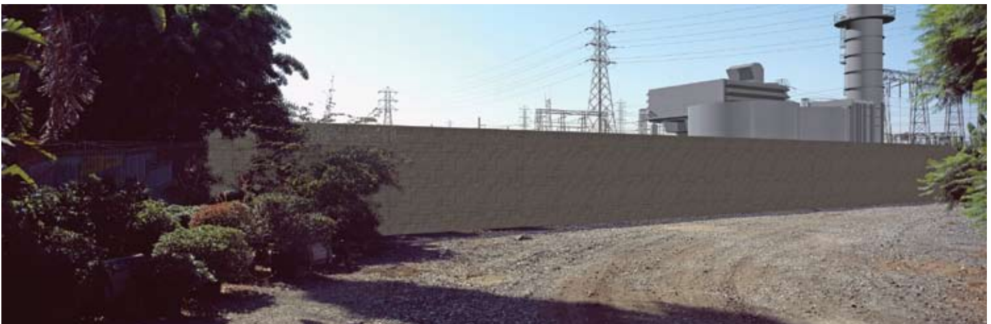
Figure 4B: Simulation of view from outside northeast corner of SCE substation facility looking southwest prior to landscaping.
