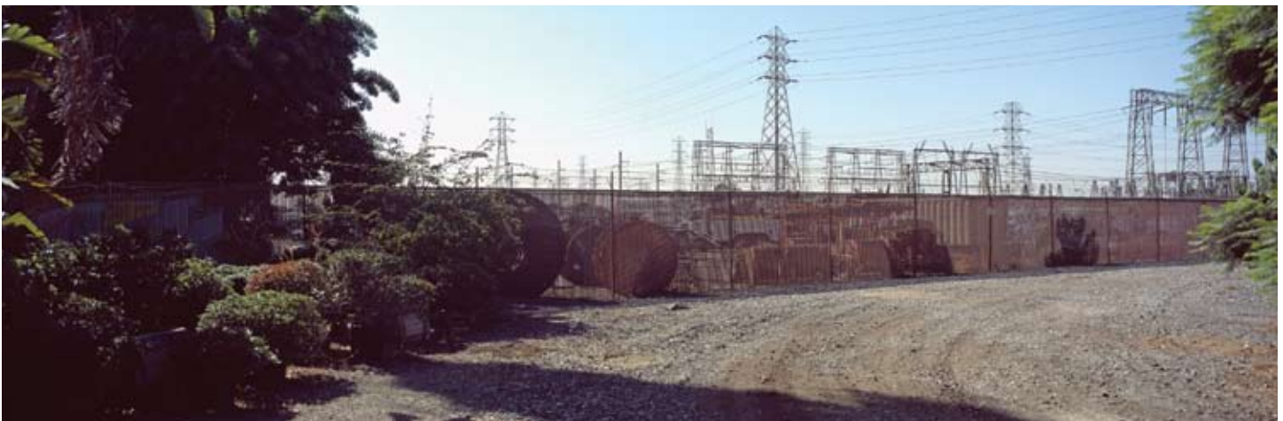
Figure 4A: Existing view from outside northeast corner of SCE substation facility looking southwest.
