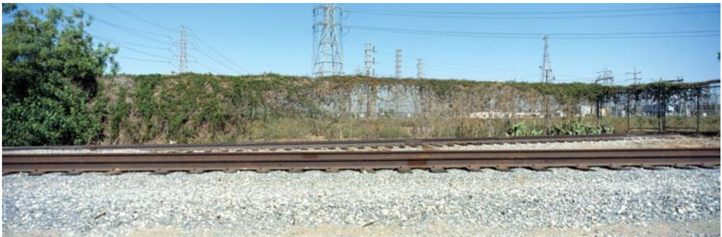
Figure 3A: Existing view from the southern border of Barre Substation, as seen from the mobile home park.
