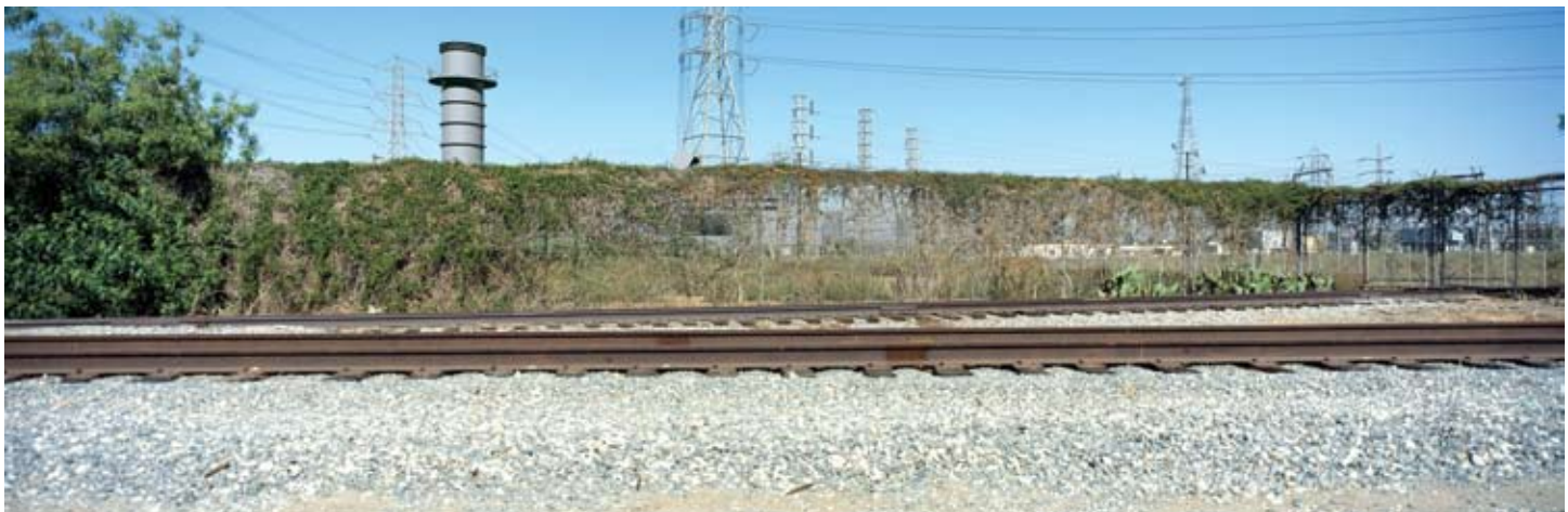
Figure 3B: Simulation of existing view from the southern border of Barre Substation as seen from the mobile home park.
