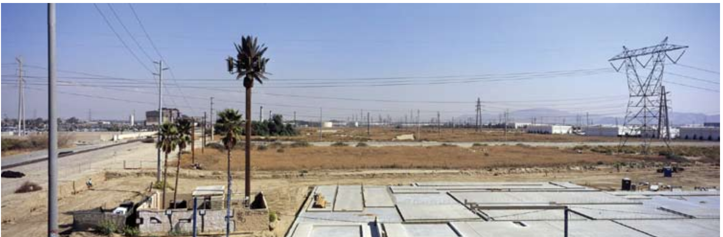
Figure 4A: Existing view of SCE property, from just east of Interstate 15 looking east
