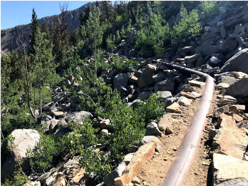
Photo 58 Access Along Pipeline
