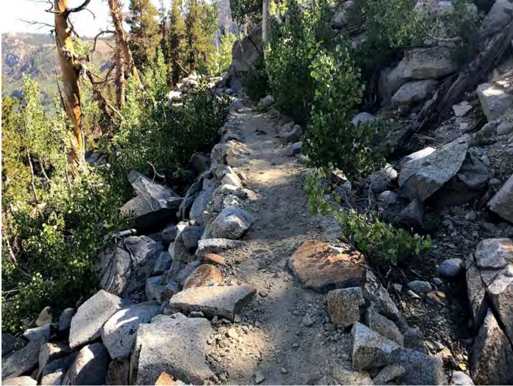
Photo 59 Access Along Pipeline
