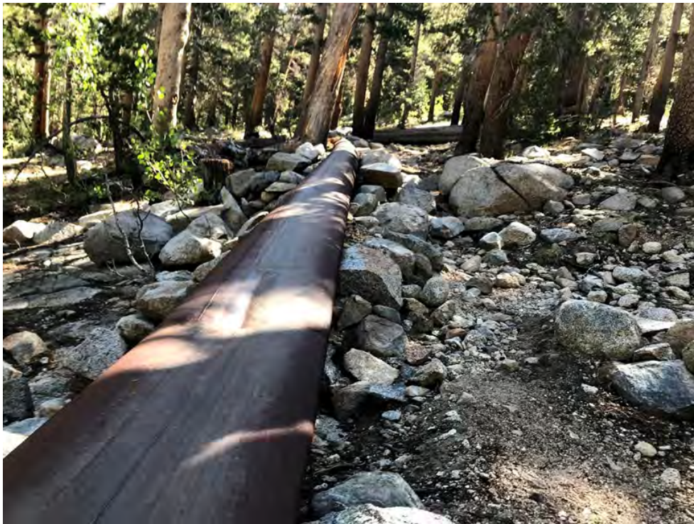
Photo 56 Access Along Pipeline
