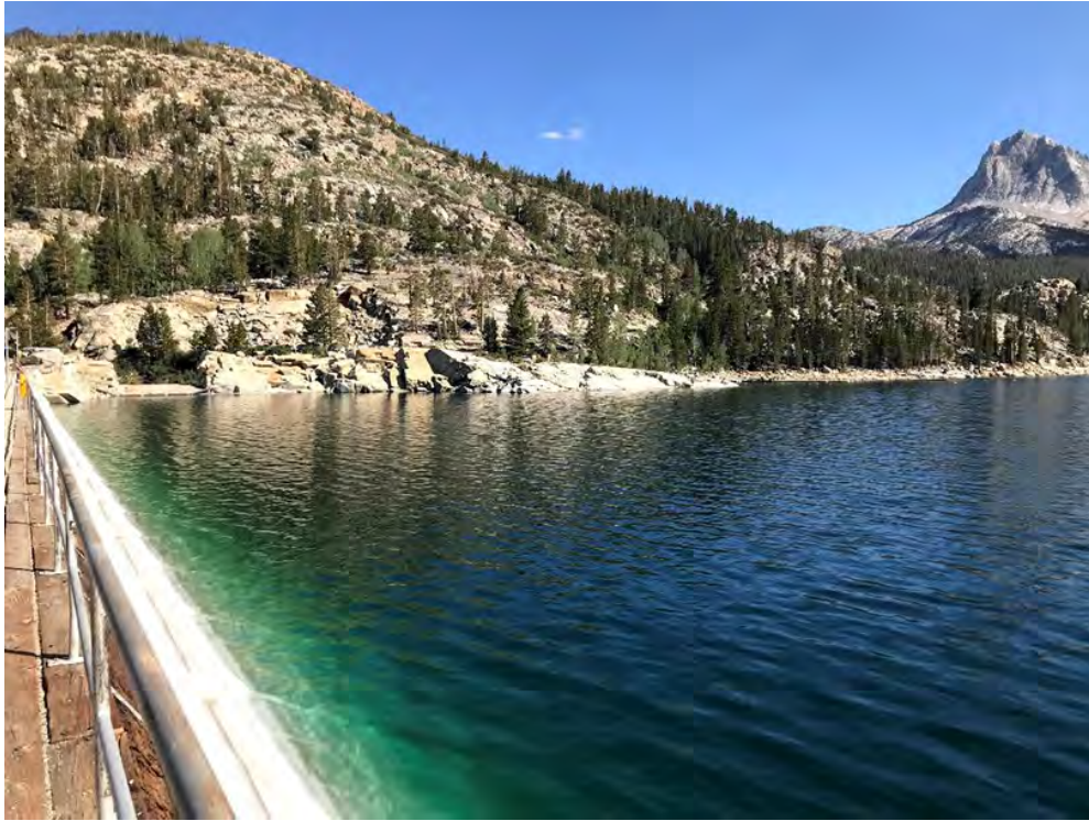
Photo 52 Upstream Face of Hillside Dam
