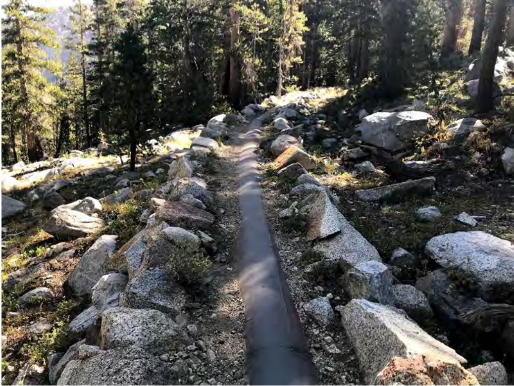
Photo 57 Access Along Pipeline
