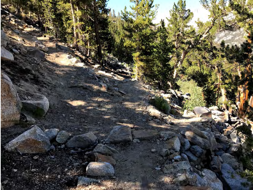
Photo 61 Pipeline Crossing USFS' Baker Summit Trail
