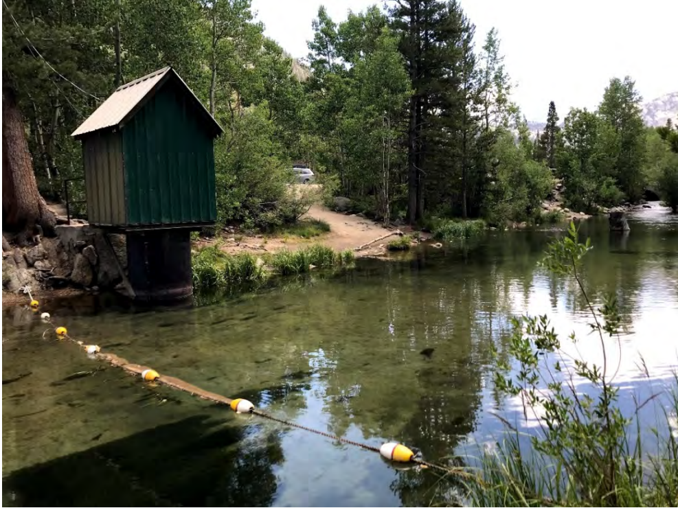
Photo 14 Shoreline Access at Weir
