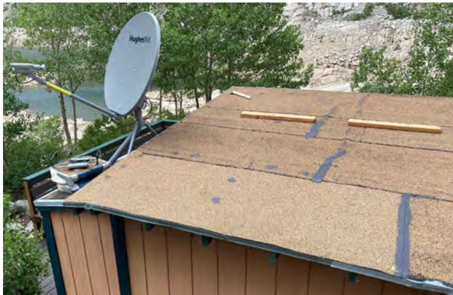
Photo 47 Roof of South Lake Landing
