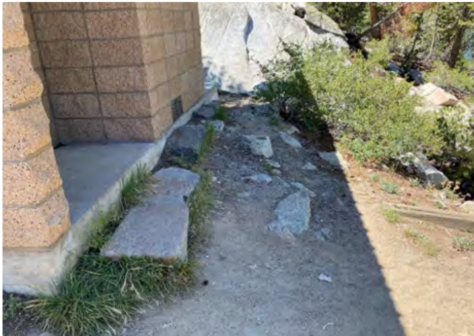
Photo 51 Bathroom Near Stairs
