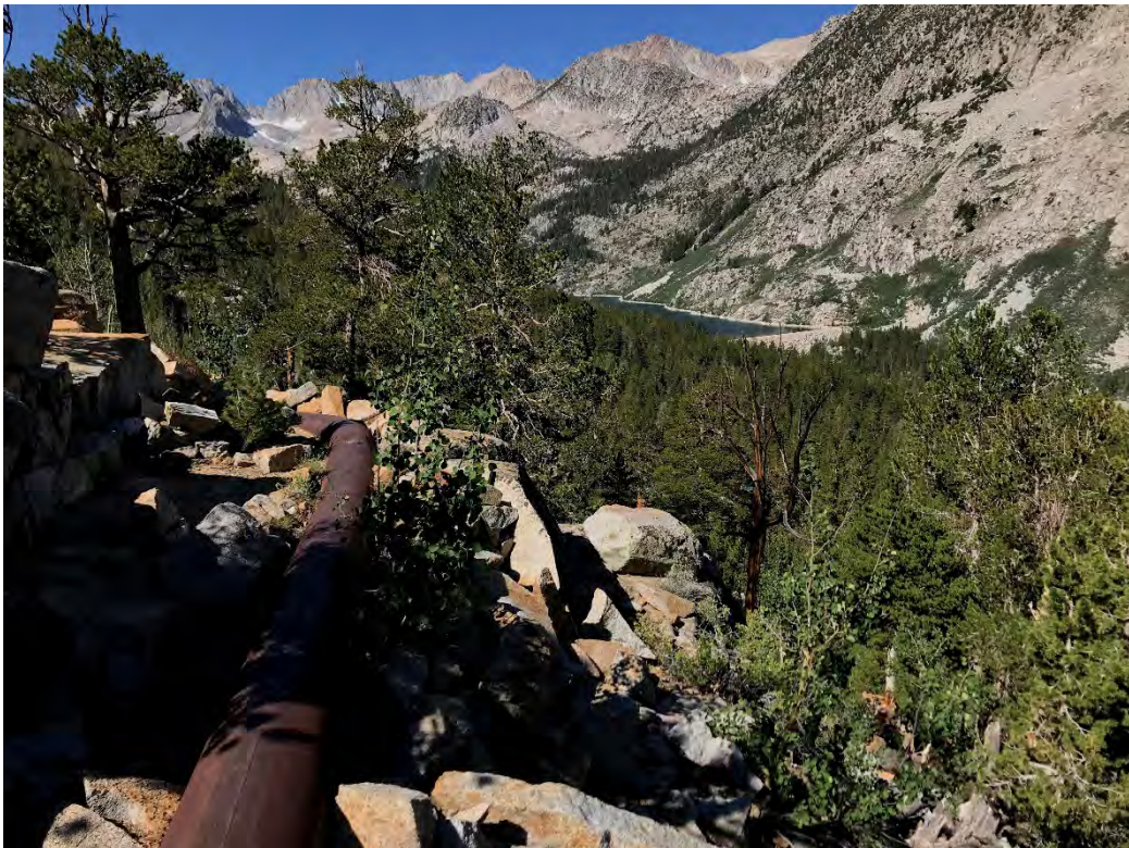
Photo 60 From Pipeline, Looking Back Towards South Lake
