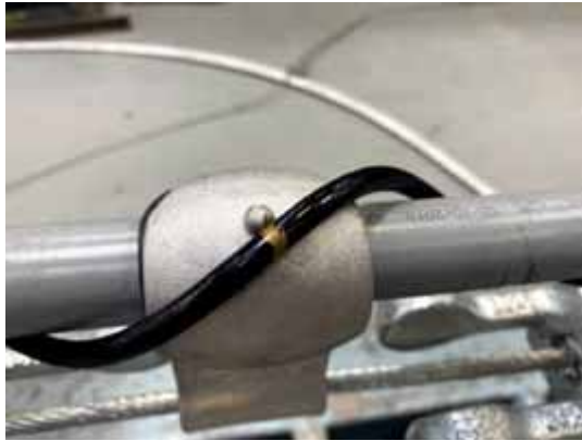
Figure CC 190–10: First Attachment Rod Placement
