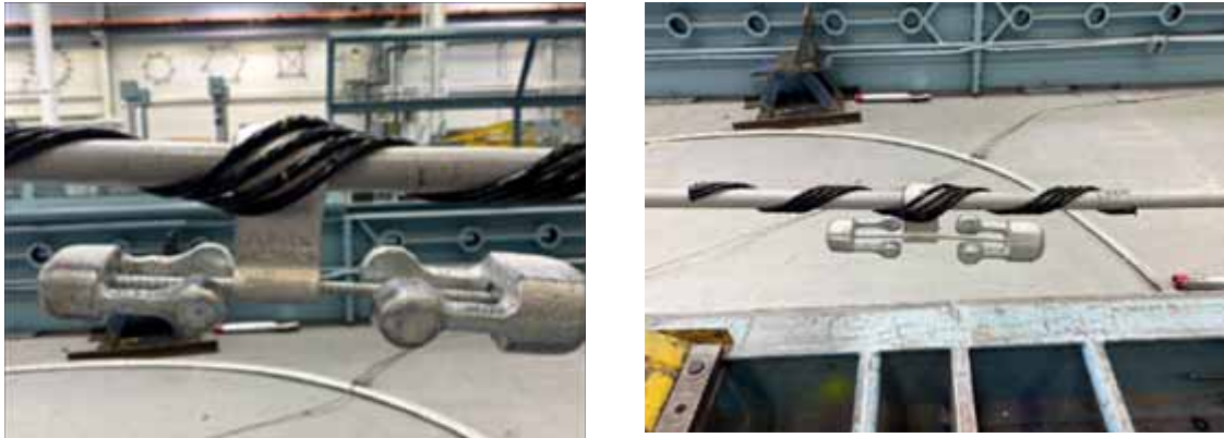
Figure CC 190–12: Completed Attachment Rod Placement
