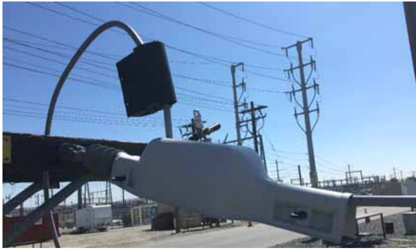
Figure CC 150-4: Connector Cover Installed at Dead-End Tap
