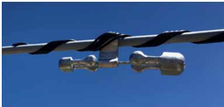
Figure CC 190-2: Stockbridge Damper
