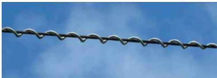
Figure CC 190-1: Spiral Vibration Damper
