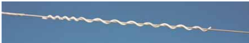
Figure 460-2: Complete Installation of Vibration Dampers
