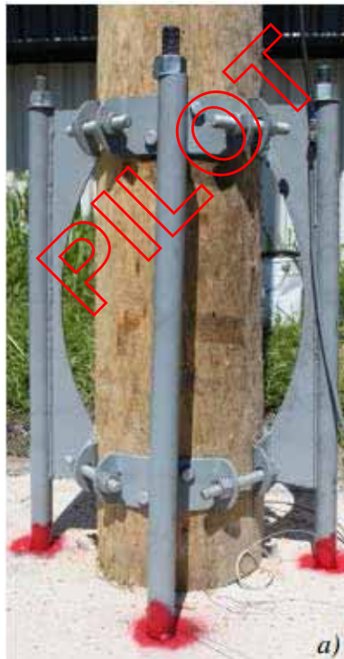
Figure PO 141P-1: Star Pole Anchor
