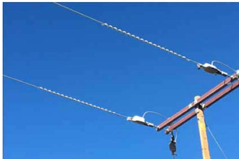
Figure CC 190–4: Installed Spiral Vibration Dampers on Covered Conductor
