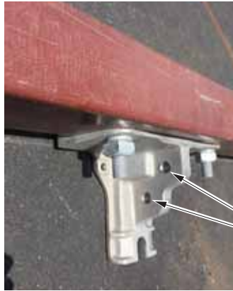
Figure PO 370–2: Composite Crossarm Mounting Bracket with Guy Attachment Holes
