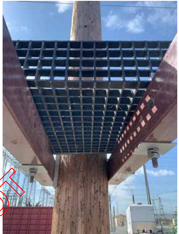
Figure DC 536P-5: Nesting Platform Top and Front View — 8-inch Bolts and 4-inch Square Washers used to Fasten Platform
