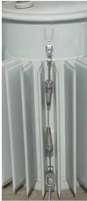
Cable Tie Down Assembly with Cable Hold-Down Roller Assembly
