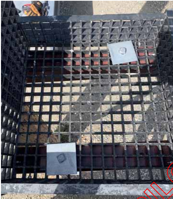
Figure DC 536P-5: Nesting Platform Top and Front View — 8-inch Bolts and 4-inch Square Washers used to Fasten Platform
