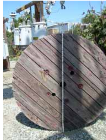
Top/Bottom of Wooden Cable Reel
