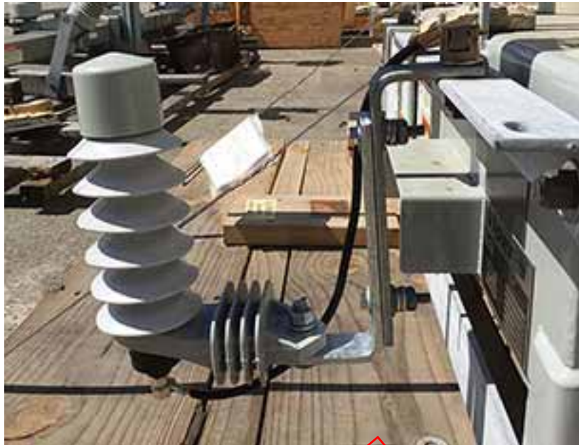
Figure IGP 100P-1: Surge Arrester Mounting Detail
