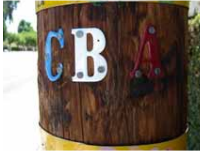
Figure PO 121-1: Pole Labeling
