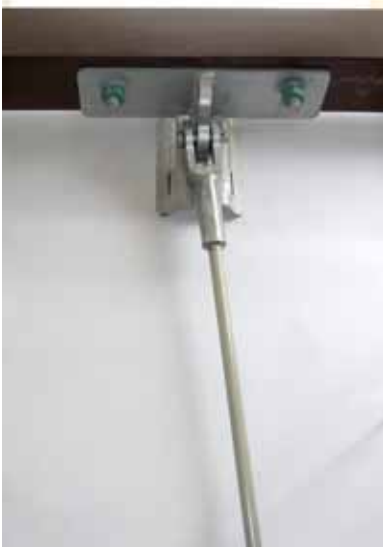
Figure PO 300–4.4: Composite Arm Dead-end Bracket
