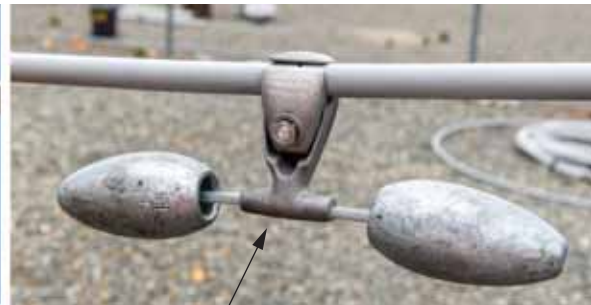
Shear Bolt Vibration Damper
