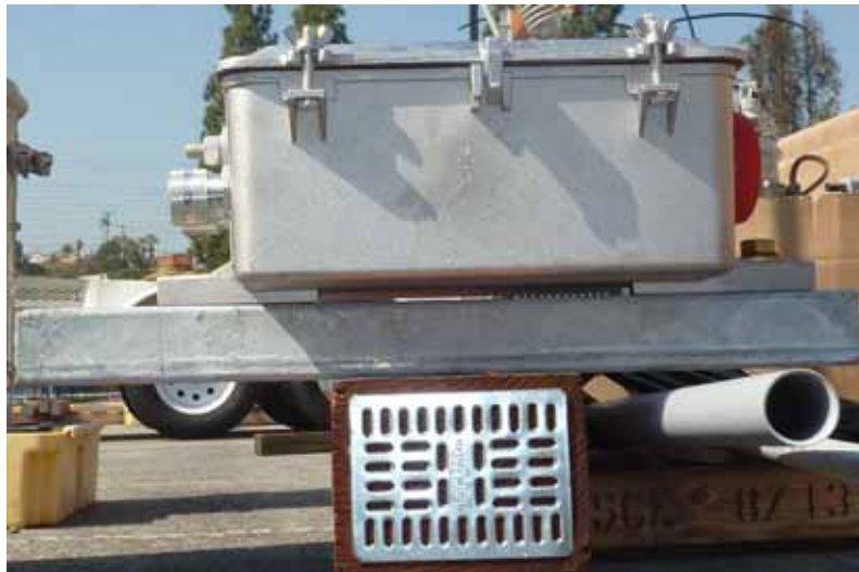
Figure SL 515-2: RCOC Relay Installation on Unistrut
