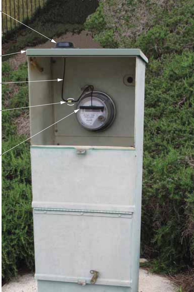
Figure T 700–6: Typical Installation Diagram for Mounting Metering Antenna to the “Top” of the Pedestal Metering Cabinet using Low Profile Antenna
