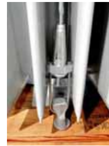
Assembly Anchored to Platform Planks
