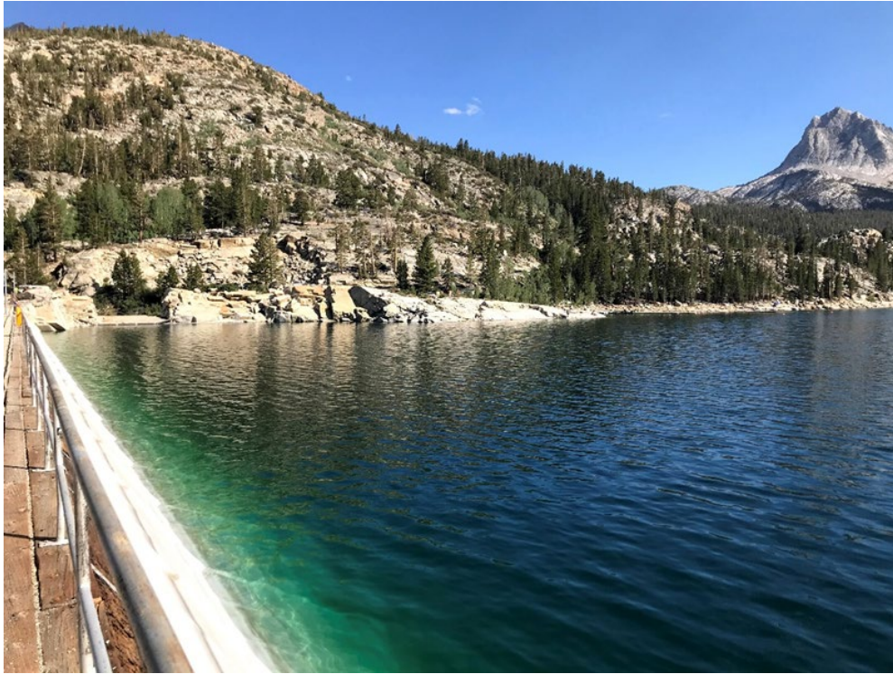
Photo 52 Upstream Face of Hillside Dam
