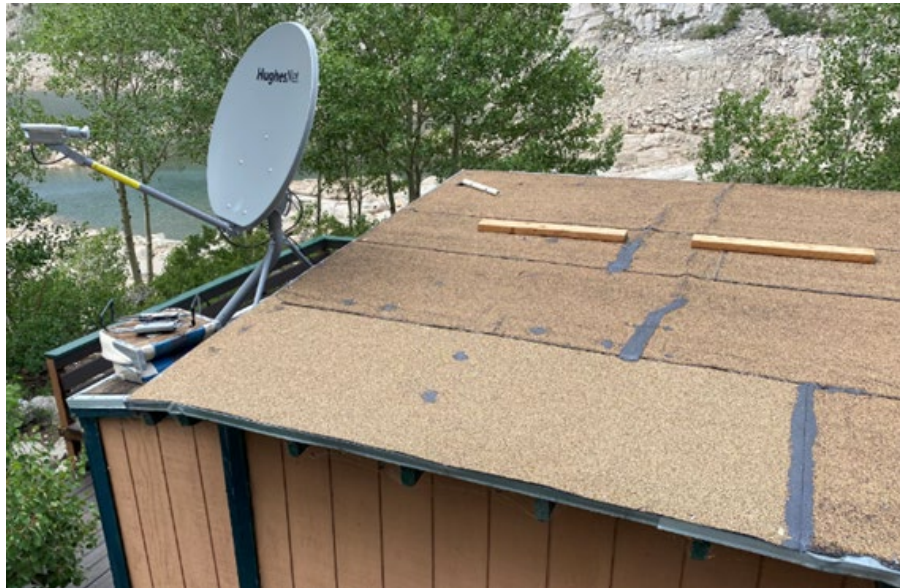
Photo 47 Roof of South Lake Landing
