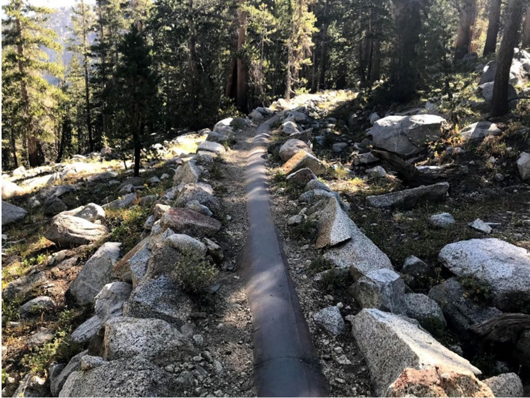
Photo 57 Access Along Pipeline
