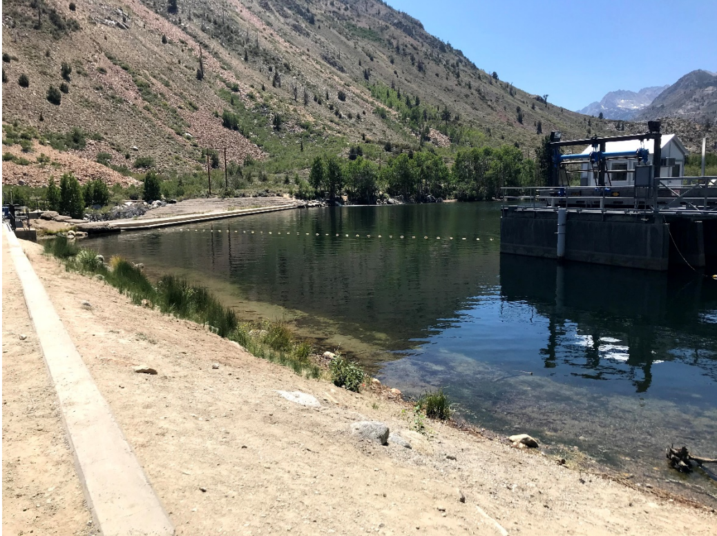
Photo 97 Access Along Intake No. 2 Dam
