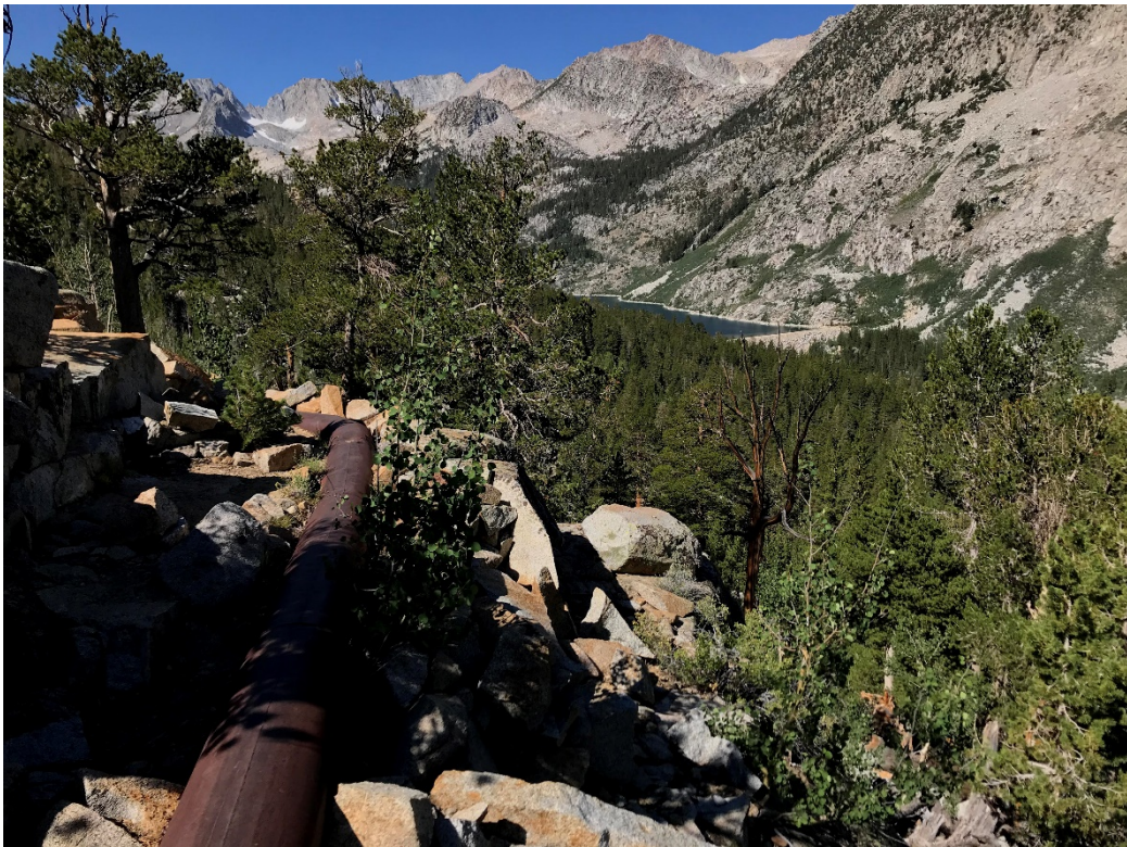
Photo 60 From Pipeline, Looking Back Towards South Lake
