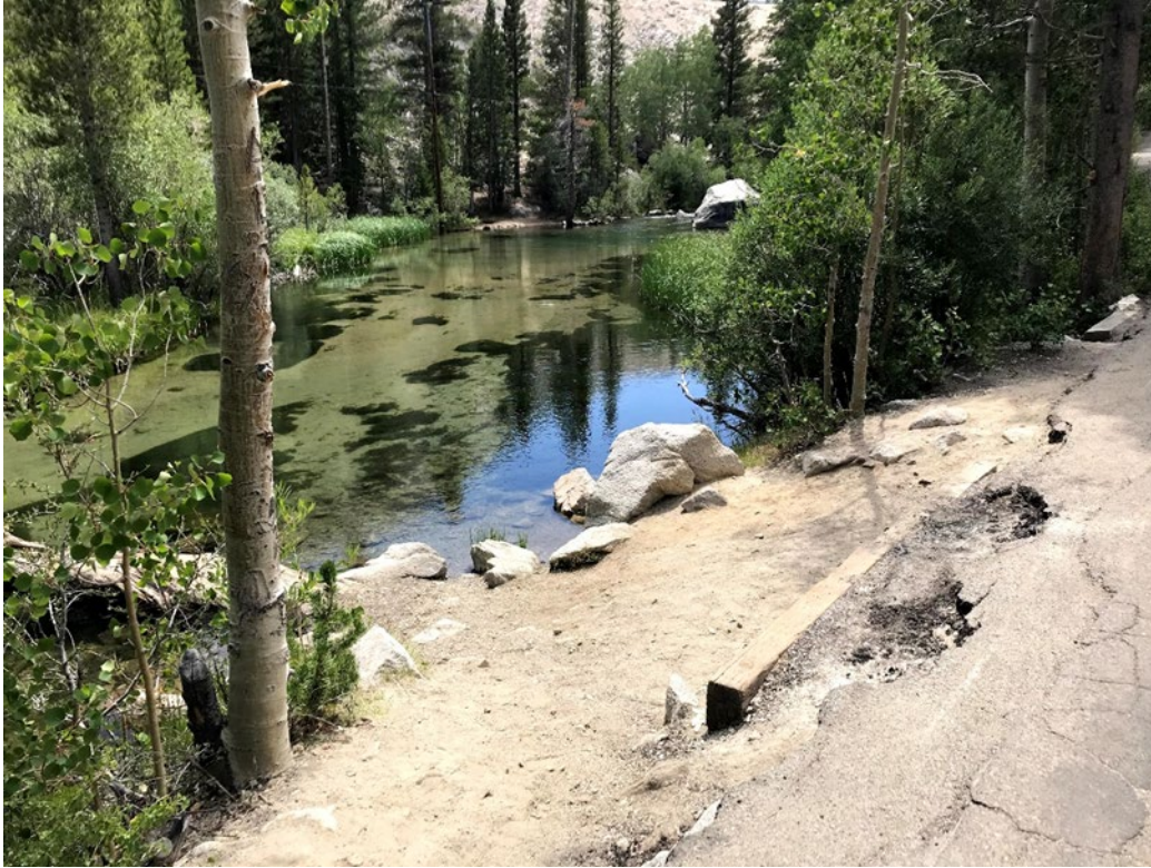
Photo 16 Access to Shoreline Upstream of Bridge
