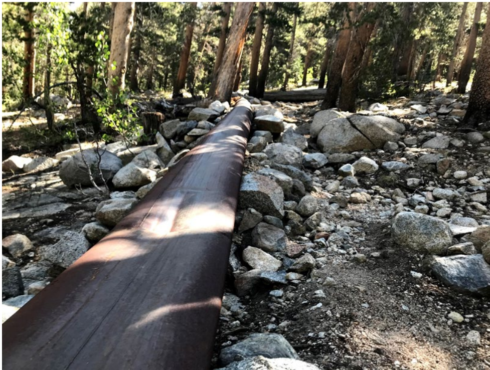
Photo 56 Access Along Pipeline
