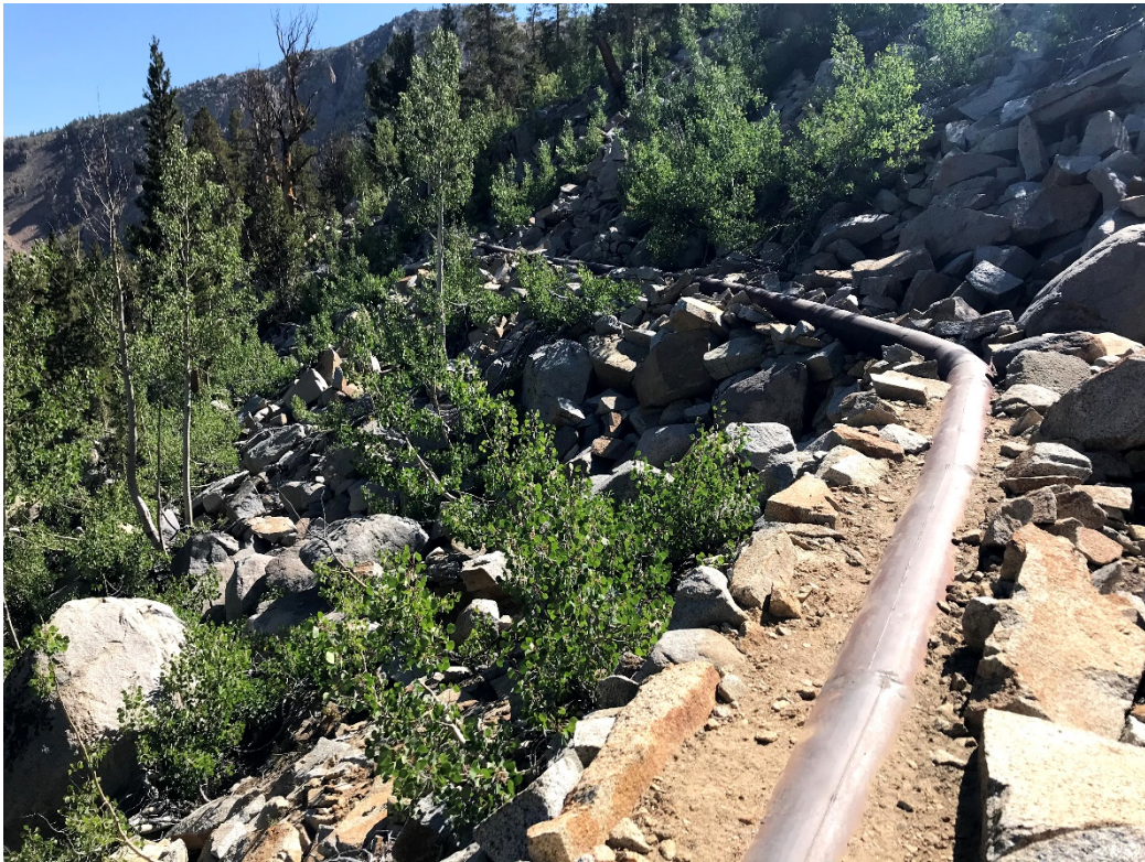
Photo 58 Access Along Pipeline
