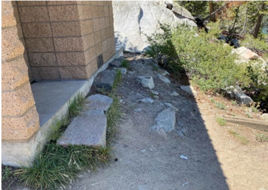
Photo 51 Bathroom Near Stairs
