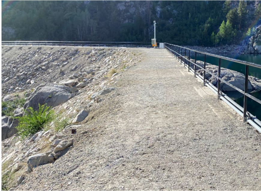
Photo 10 Crest of Sabrina Dam
