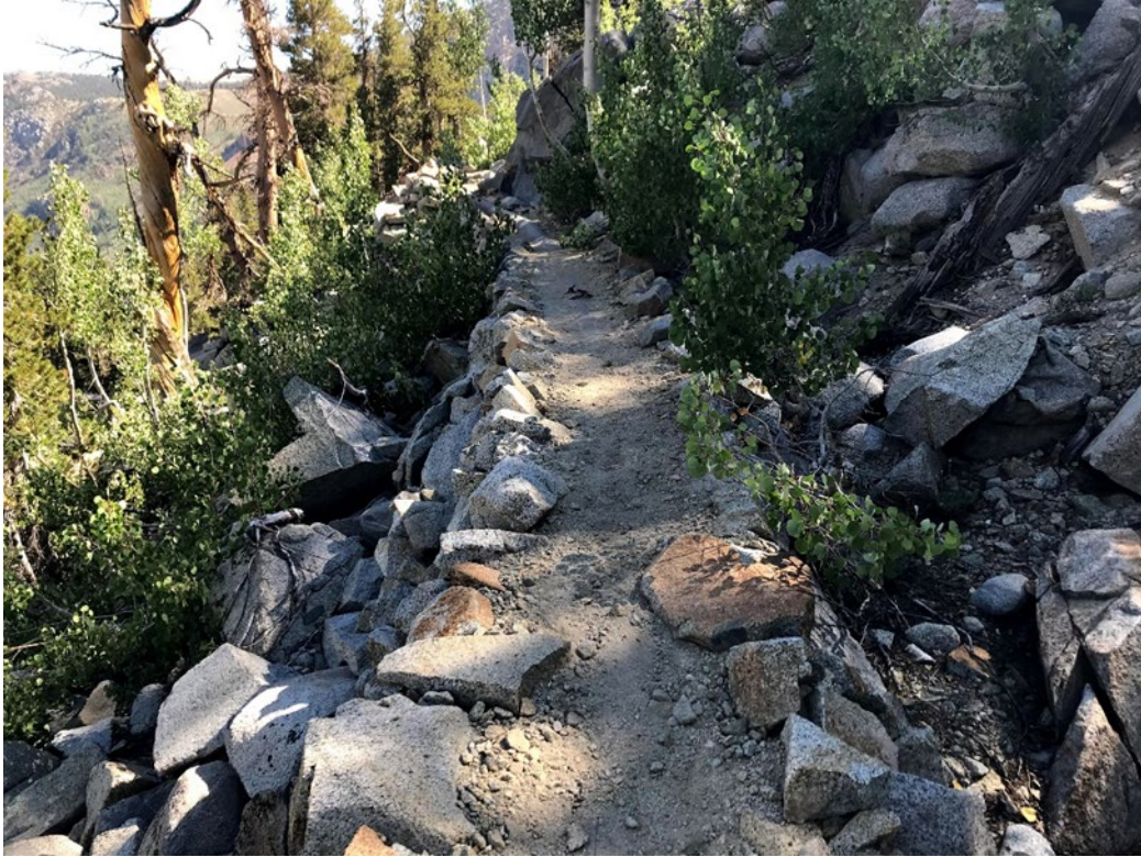
Photo 59 Access Along Pipeline
