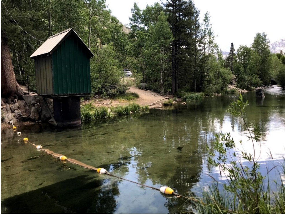
Photo 14 Shoreline Access at Weir
