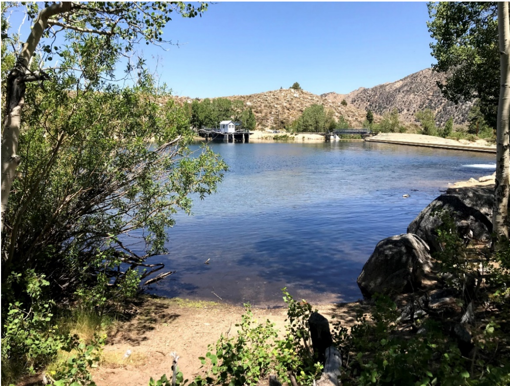
Photo 111 Access to Shoreline
