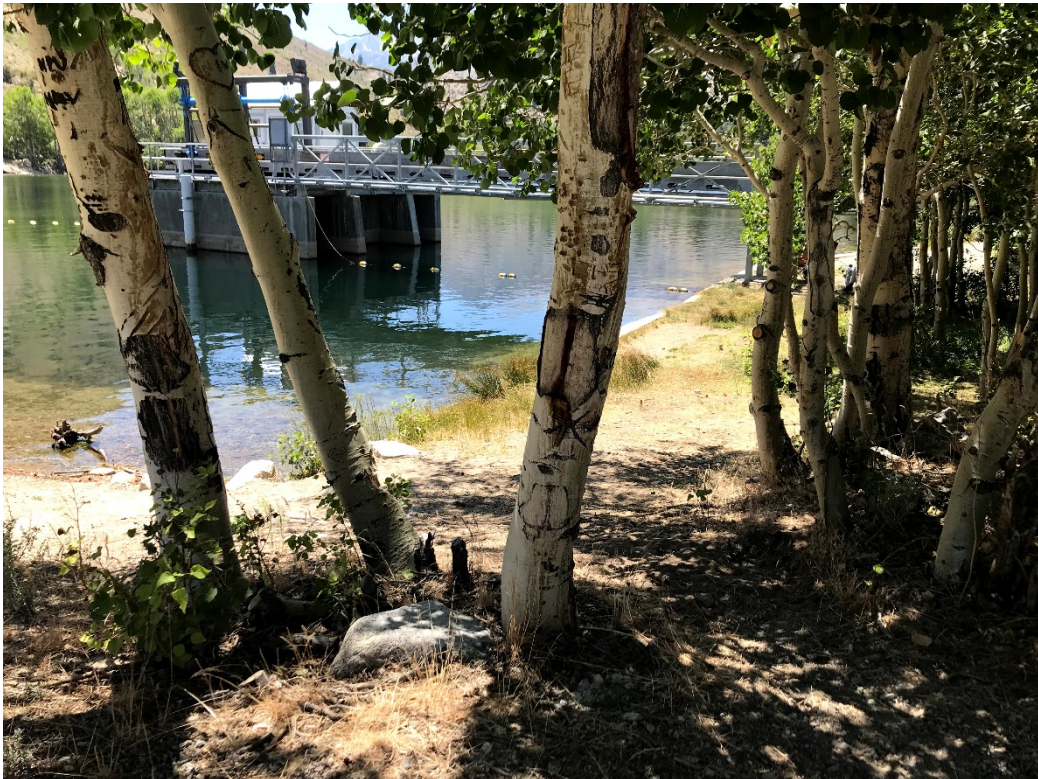
Photo 96 Access Behind Intake
