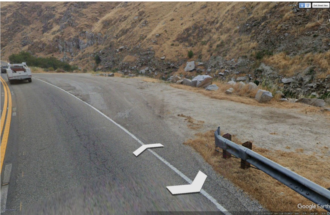
Photo 8. Looking south at River Site 4 parking area; space for approximately 6-10 vehicles in this dirt turnout on the north side of SR 178.
