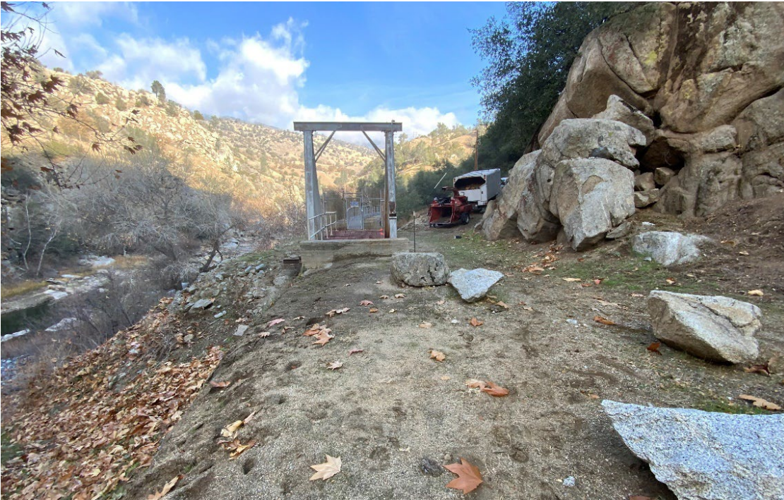
Photo 11. Democrat Gage Trail, proposed trailhead monitoring location. Note this monitoring location is located approximately 0.95 miles southwest from SR 178, along an existing paved access road (Democrat Dam Road) with no public vehicle access (locked gate).
