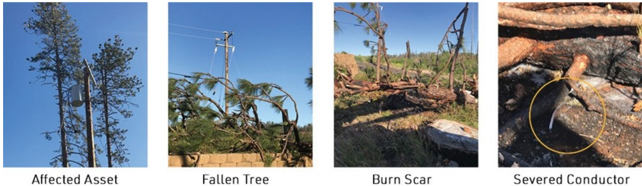
Figure CC-2 PG&E Covered Conductor Effectiveness – Example 1
