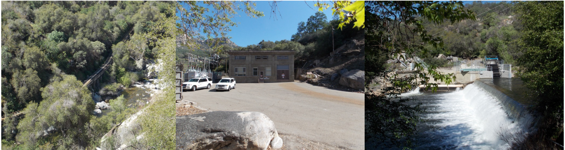
Middle Fork Kaweah River Kaweah No. 3 Flume
