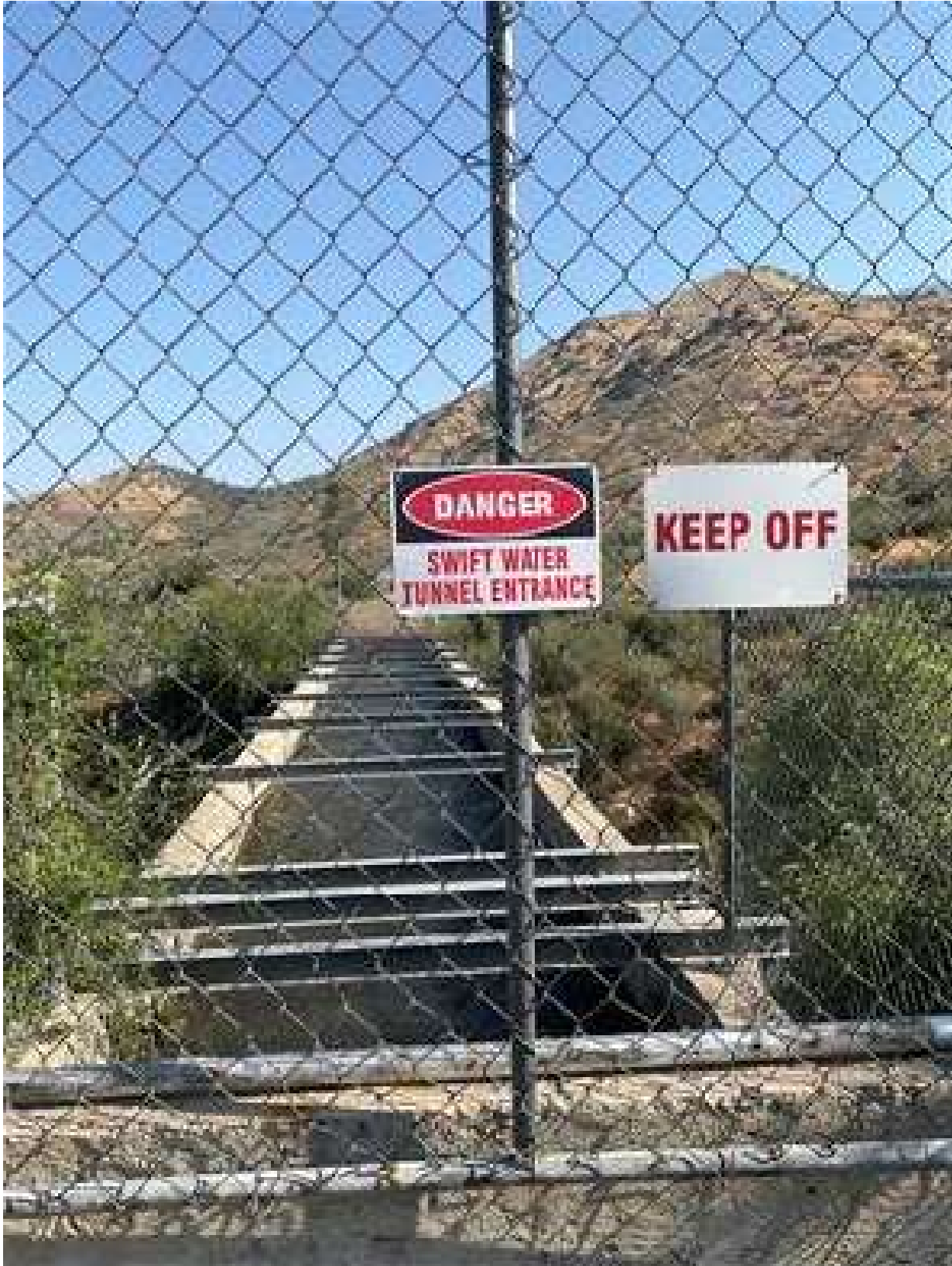
Tunnel at 18 Corral Creek Access (002).jpg
