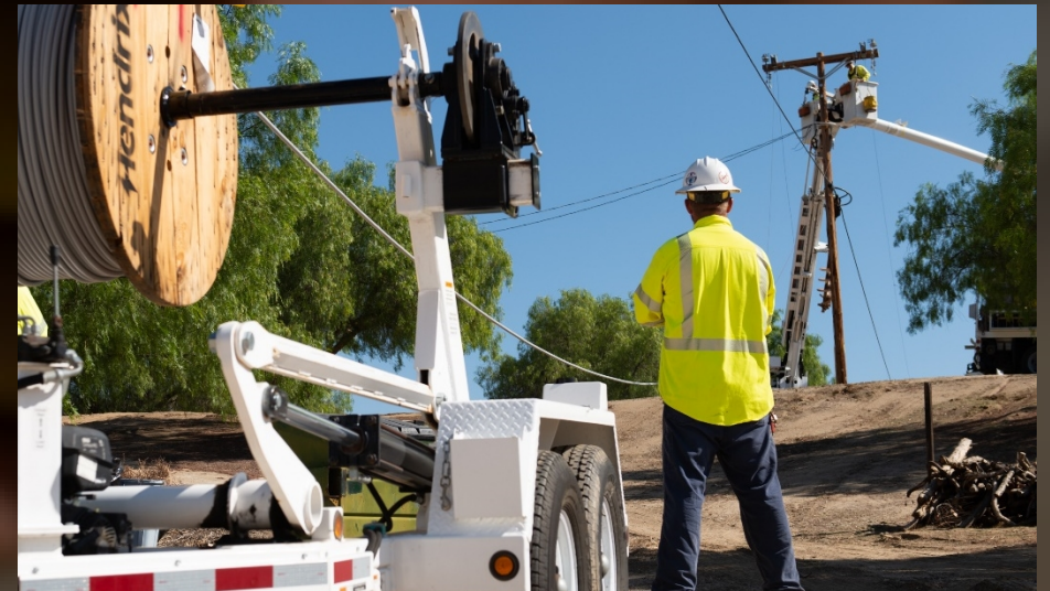
Above photos: SCE crew installing insulated wire
